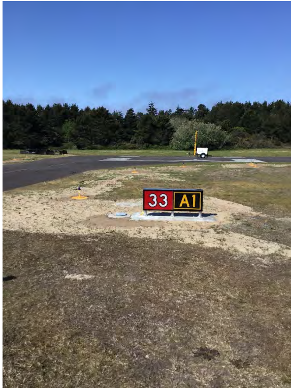
Guidance Sign Installation
