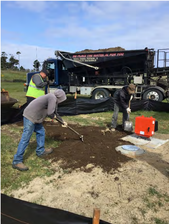
Topsoil Placement
