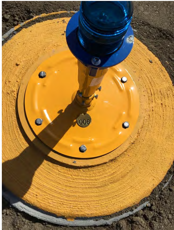
Light Identifier Tags Installed
