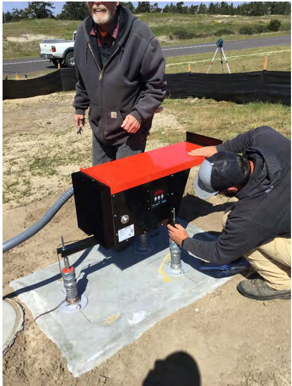
Runway 15 PAPI Installation
