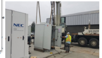
EWEB contractor installs back-up battery power system.
