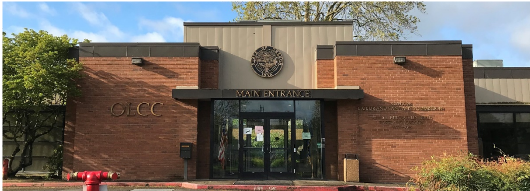
OLCC Headquarters – McLoughlin Blvd.
