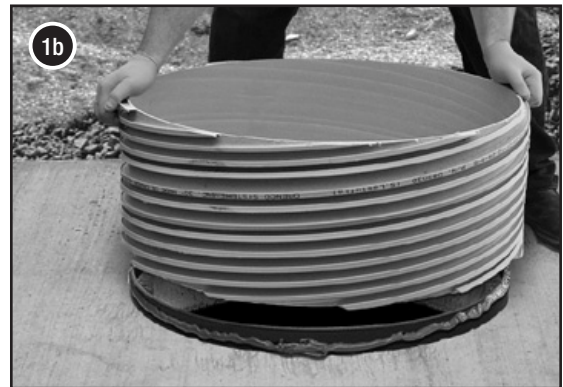
Install access riser
