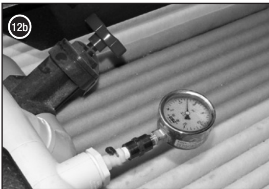
Install pressure gauge
