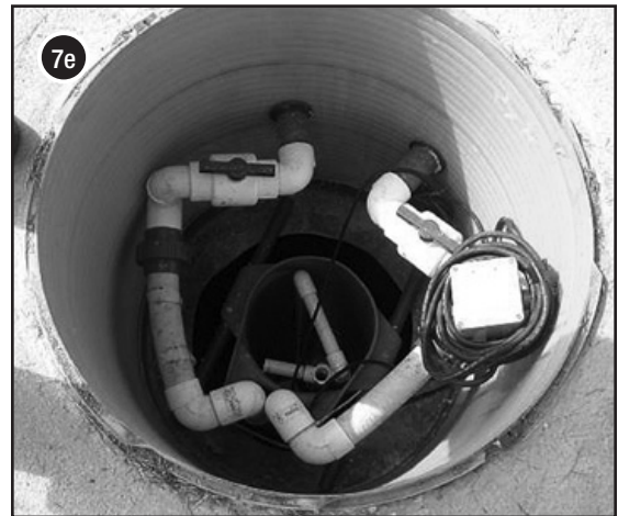
Orient discharge assemblies for ease of maintenance
