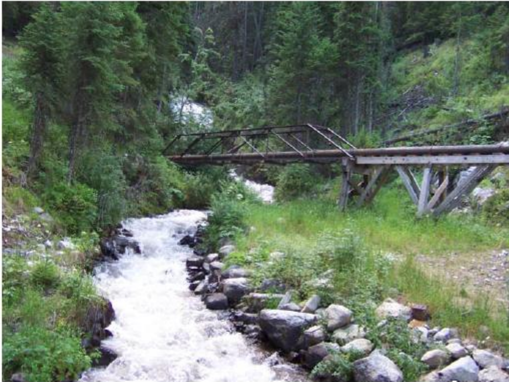
Figure 10: Project penstock crossing over by-passed reach of East Fork Wallowa River. (PacifiCorp, 2011)
