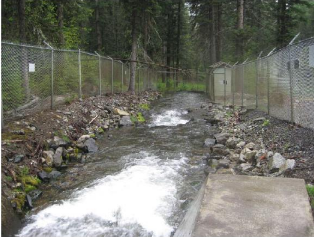
Figure 12: Project Tailrace looking downstream from Powerhouse. (PacifiCorp, 2011)
