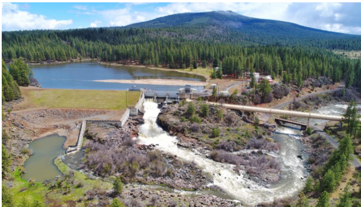
Figure 5: J.C. Boyle Dam
