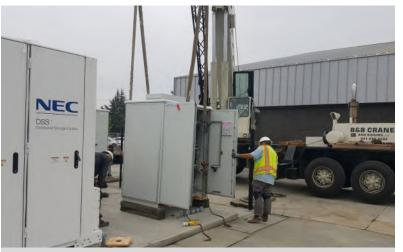
EWEB contractor installs back-up battery power system.
