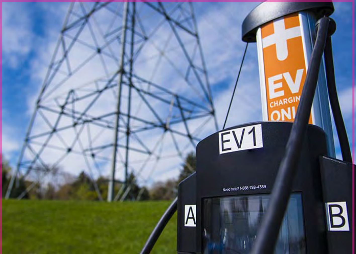
EV Charging pedestal in front of electricity transmission lines. Photo source: betterenergy.org
