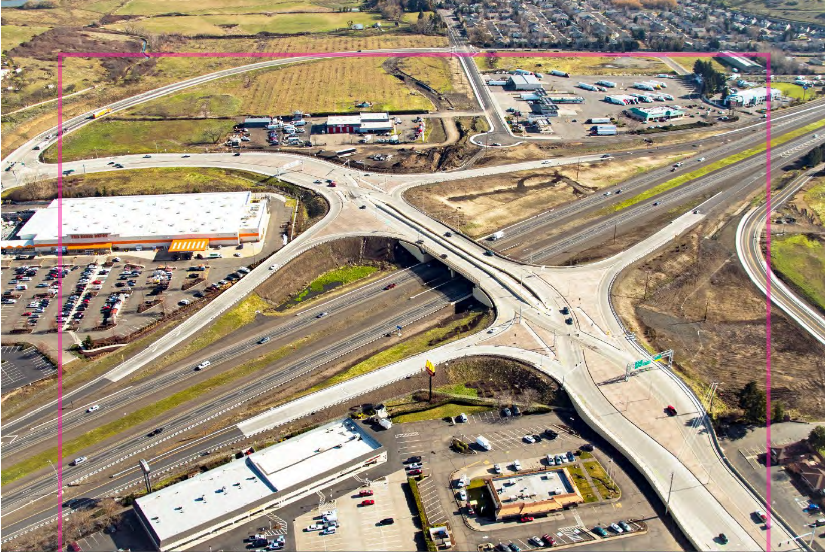
I-5 Fern Valley Interchange, Phoenix, Ore., Photo credit: ODOT via Flickr
