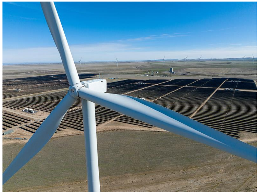
Wheatridge Energy Facilities, Morrow County Photo: Portland General Electric
