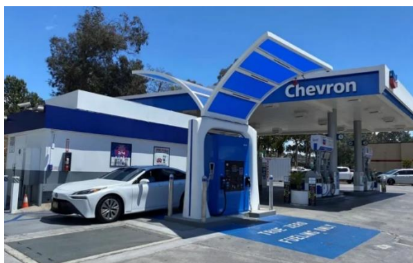
Hydrogen refueling station in Berkeley, CA.
