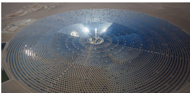
Concentrating solar-thermal power plant. Photo: U.S. Department of Energy
