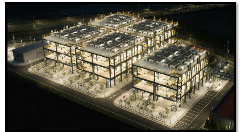
Hanwha Energy Hydrogen Fuel Cell Plant, Daesan, South Korea. Source: Koreaherald.com.
