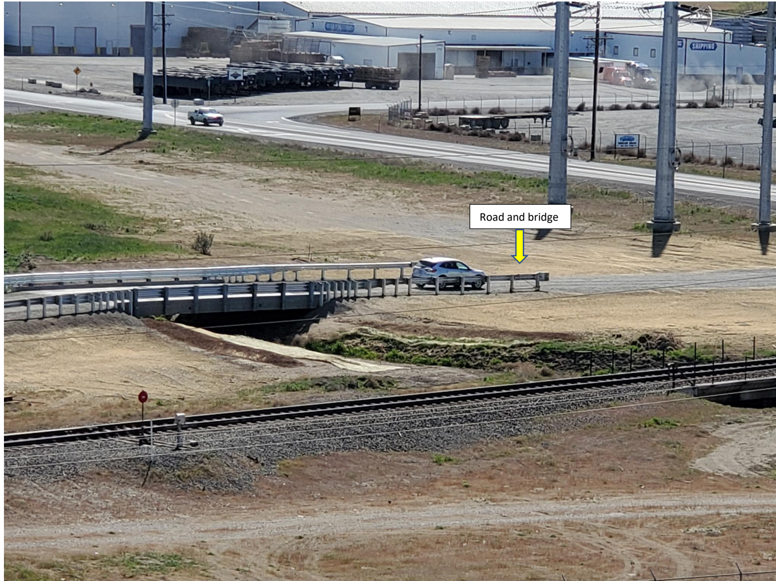
Figure 3: Perennial Wind Chaser Station – Road and Bridge (Current Conditions)
