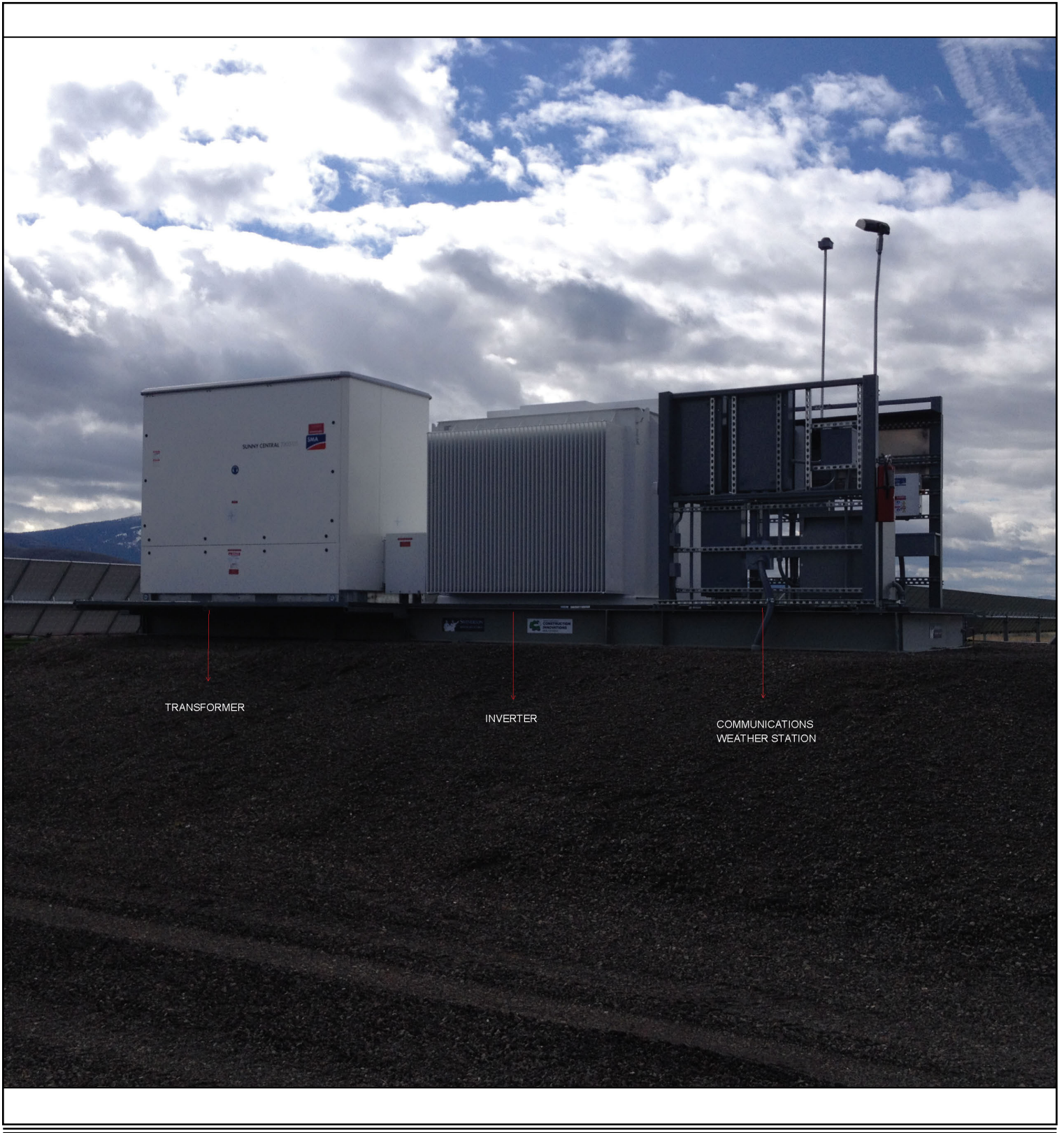
Figure B-7 Illustration of Inverter/Transformer Installation
