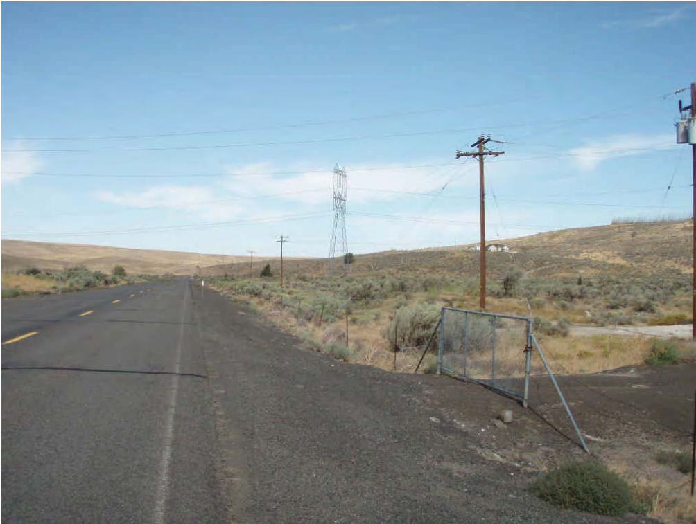
Photo 5: KOP 4 - SR74 Looking North at Existing PGE Transmission Line
