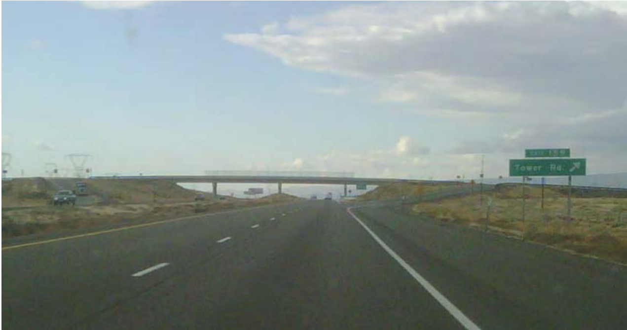
Exhibit 2 I-84 Westbound, Tower Road Exit No. 159
