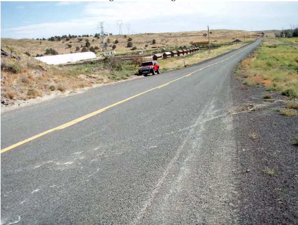
Photo 4: KOP 3 - SR 74 Looking South at Existing PGE Transmission Line
