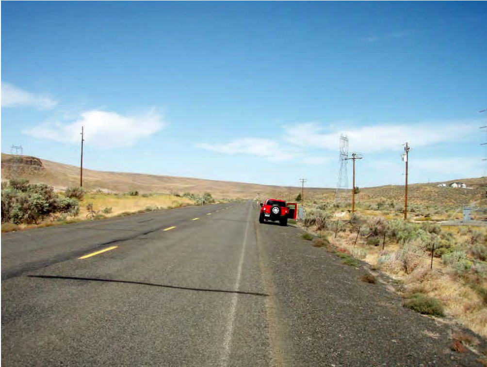
Photo 3: KOP 2 - SR 74 Looking North at Existing PGE Transmission Line
