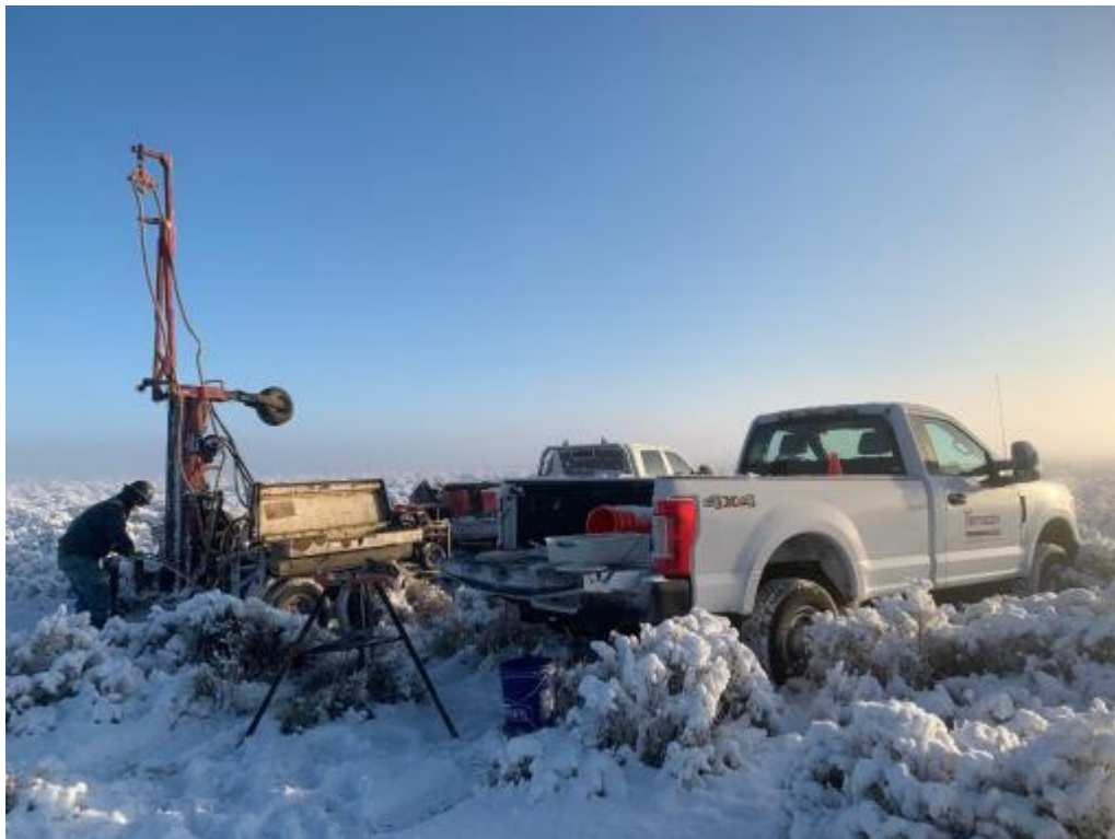
Photo 4: Drilling activities at project site
