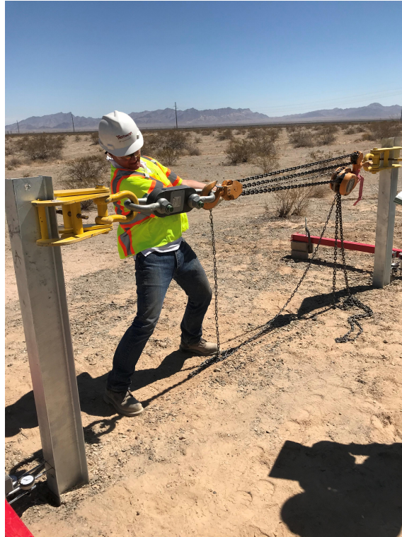
Typical Photo of Load Cell Connected to Two Test Piles.
