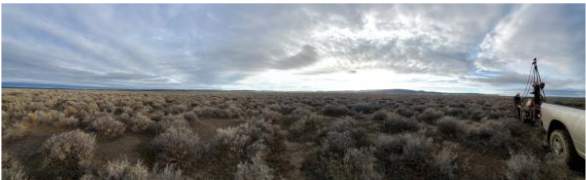
Photo 2: Drilling activities at project site
