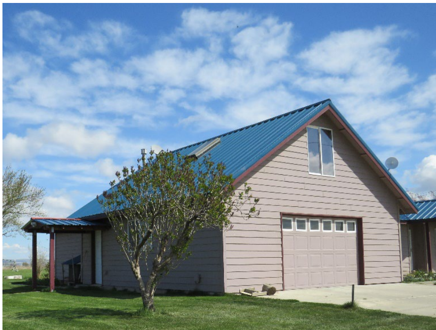
Photograph 4. 79023 Melody Ln., Stanfield, OR. View to the Northeast.
