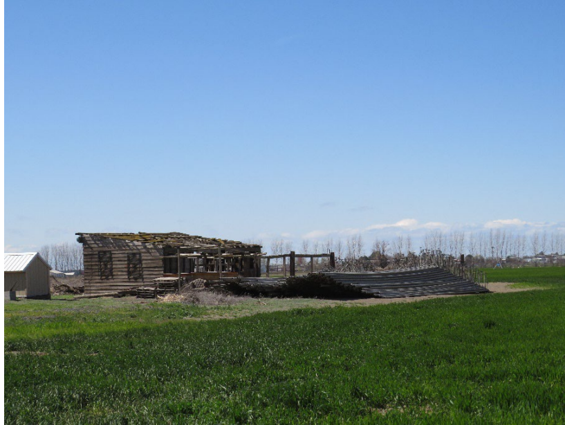
Photograph 8. 78926 Melody Ln., Stanfield, OR. View to the Southwest.
