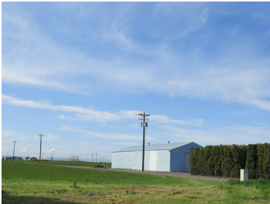
Photograph 2. 32548 E Highland Ext., Stanfield, OR. View to the Southwest.
