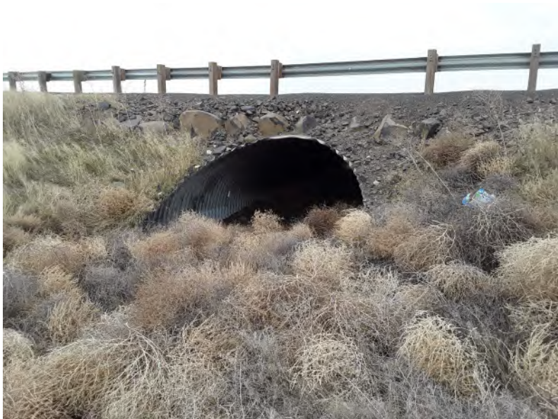
Photo 87. Culvert on EPH-02B. Looking SE. 3/8/2021.
