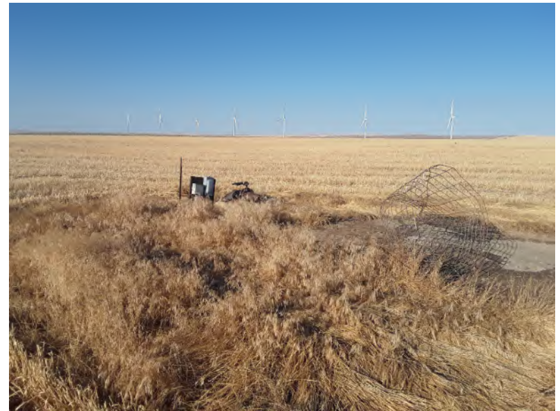
Photo 4. Abandoned pipeline shows as visible dark spot in some orthoimagery. Looking SW. 7/27/2020.
