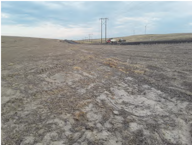
Photo 31. EPH-01 no longer has channel. Looking NE. 7/28/2020.
