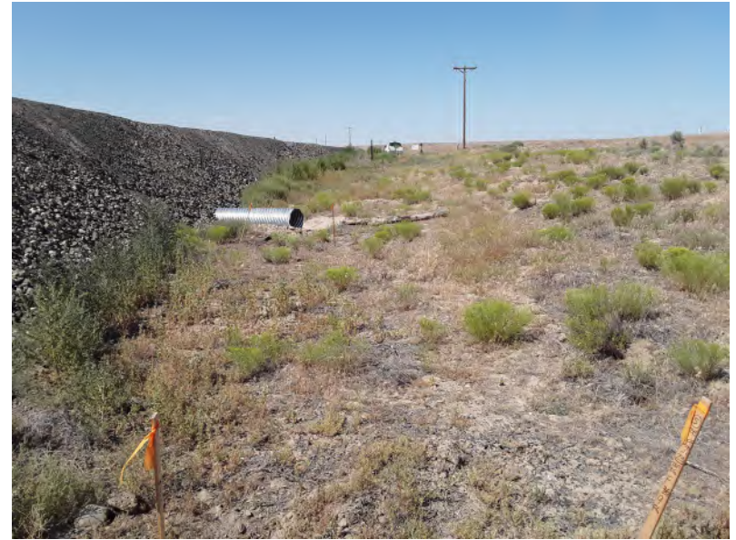
Photo 26. Newly installed culvert, no bed or banks. Looking W. 7/27/2020.
