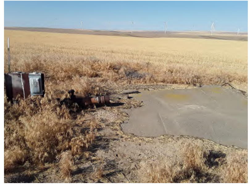
Photo 18. Dark spot on orthoimage. Looking SW. 7/27/2020.
