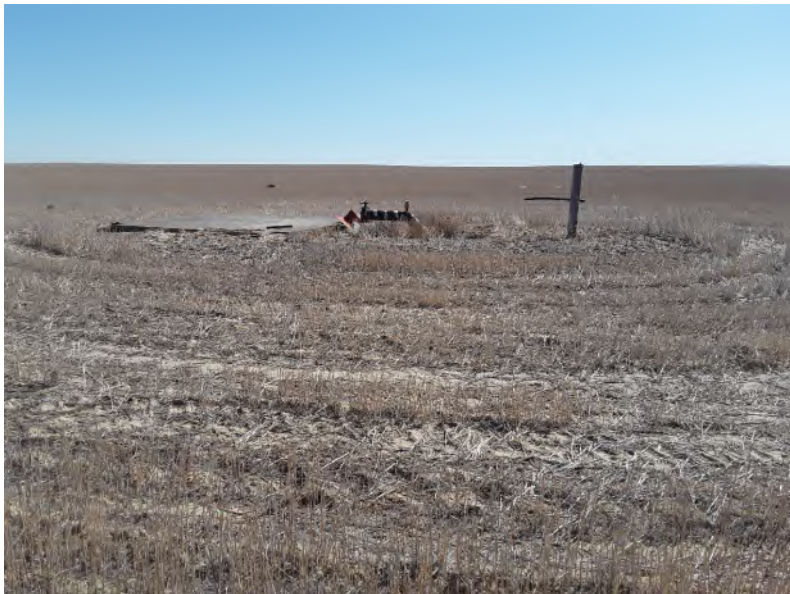
Photo 11. Abandoned pipeline shows as visible dark spot in some orthoimagery. Looking NE. 7/27/2020.
