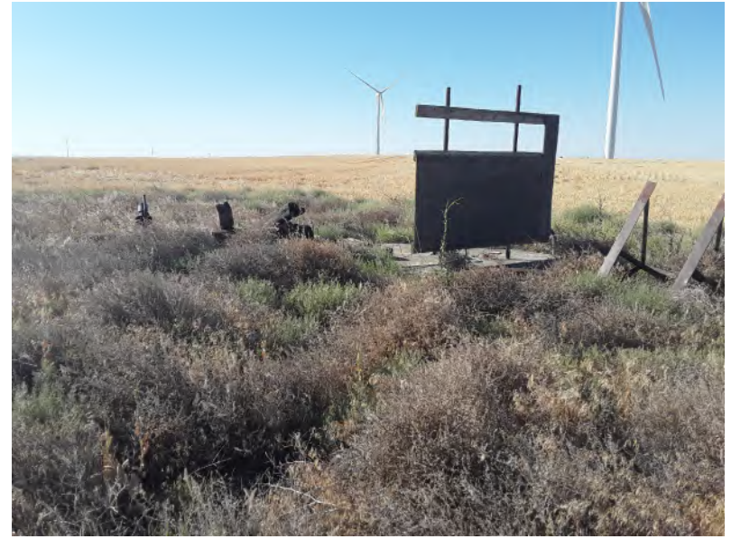
Photo 6. Abandoned pipeline infrastructure shows as visible dark spot in some orthoimagery. Looking SE. 7/27/2020.
