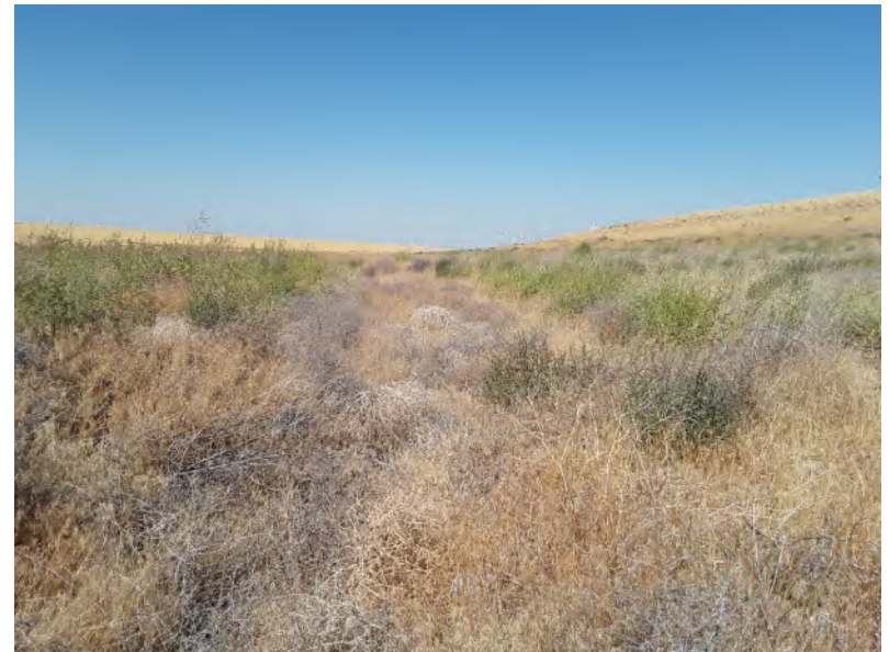
Photo 96. Ephemeral stream drainage (EPH-05). Bed and banks buried under Russian thistle. 1 foot wide. Looking N. 9/13/2021.
