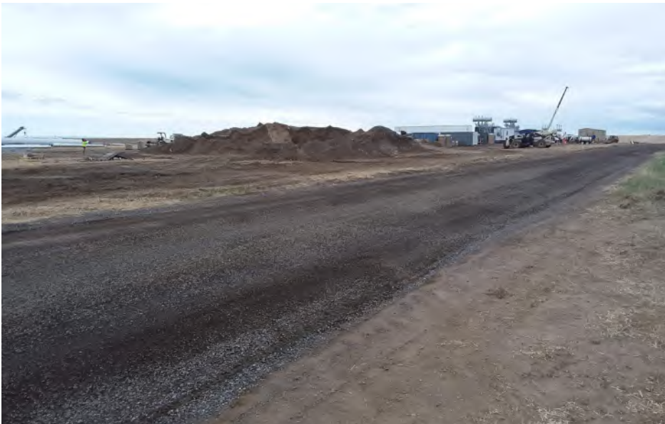
Photo 3. Category 6, Developed-Other. Substation construction.
