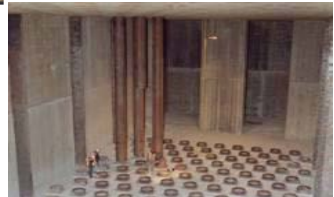
Vault under construction
