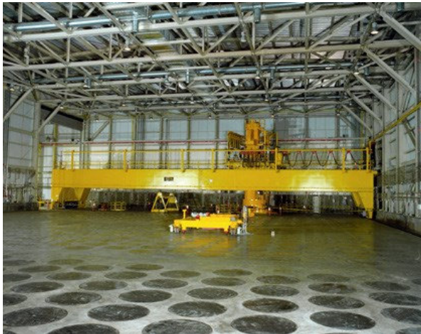
Circles in facility floor are locations of storage tubes (CH2M 2016)
