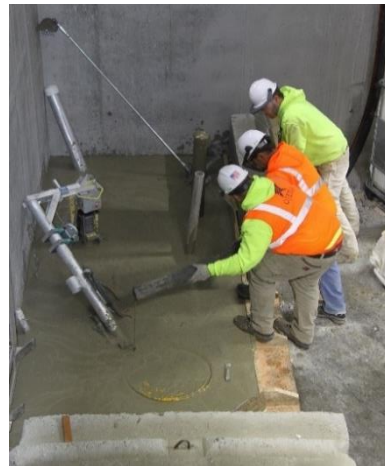
Grout and debris added at mock-up to simulate B-Cell flooring
