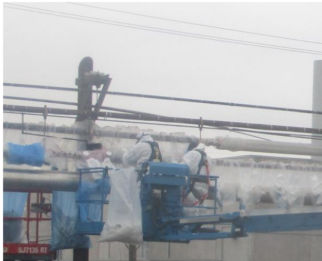
Workers removing asbestos-clad steam lines
