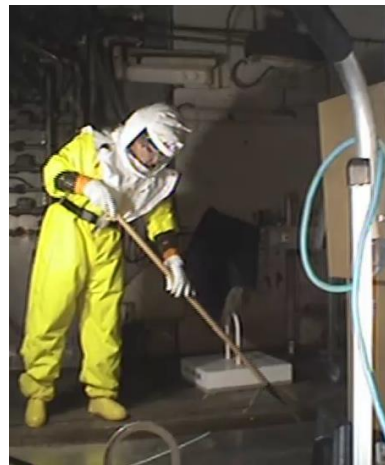
Radiological cleanout of airlock trench
