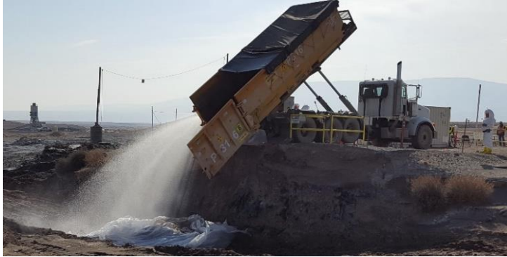
Disposing of debris at Environmental Restoration Disposal Facility
