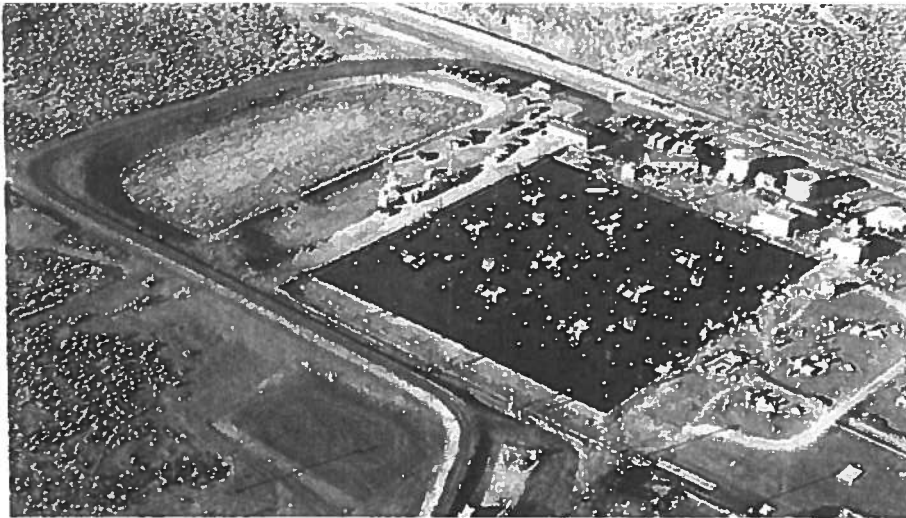
At center are the new interim surface barriers at the SX Tank Farm.
