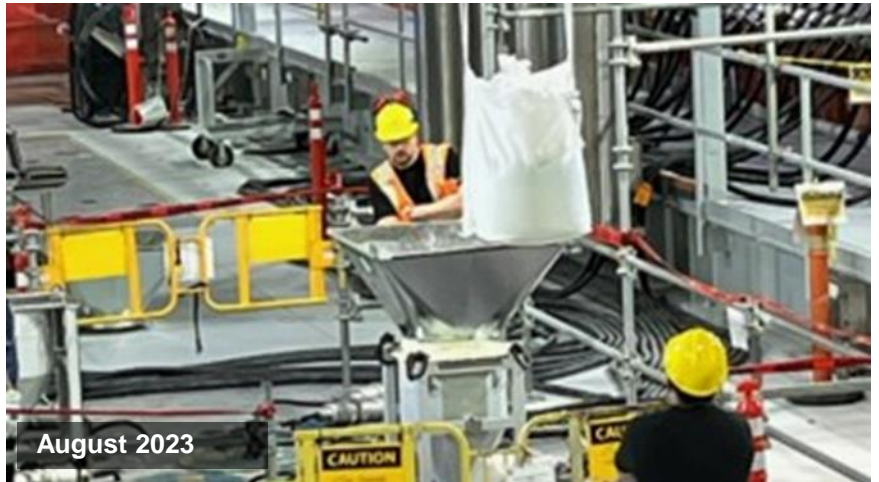
First bag of frit being poured into Melter 1
