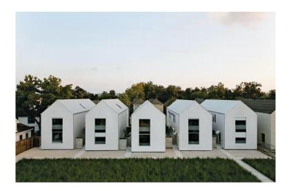
Allowing zero-lot line builds doesn't mean all developments will fill that lot width fully. This is an example of houses built about 5 feet apart rather than the standard 10 feet created by 5-foot side yards.
