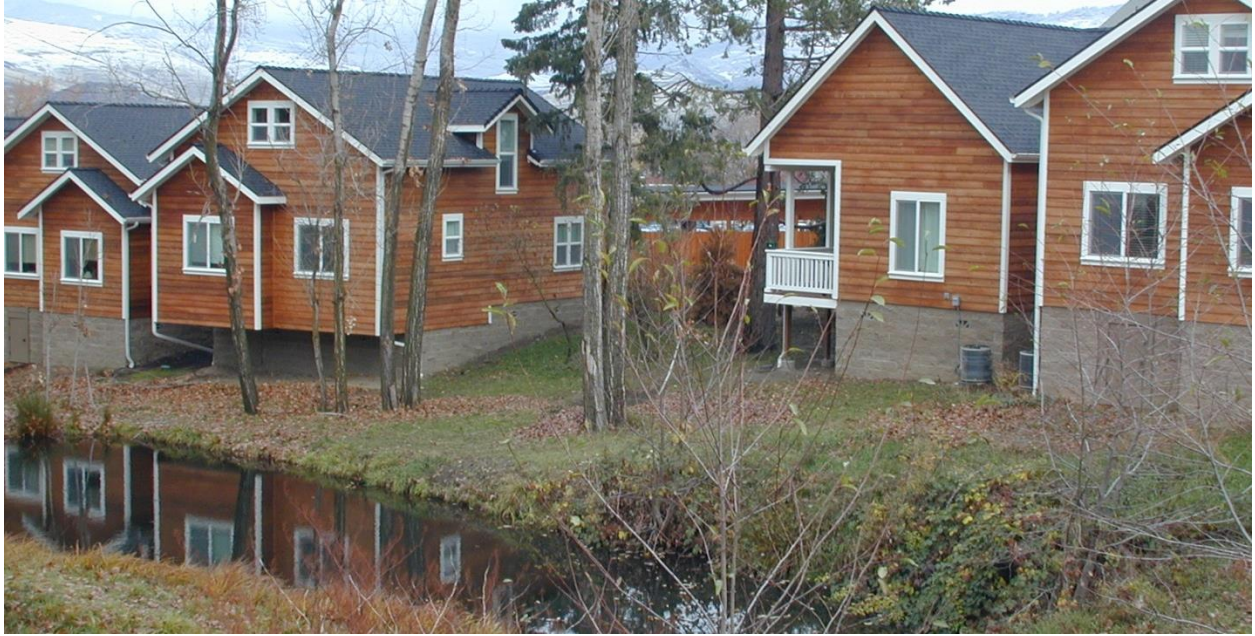
Figure 35. Ashland Creekside Housing.
