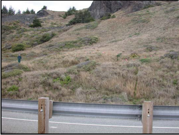
Figure 10. Meyers Creek site, viewed from across Highway 101
