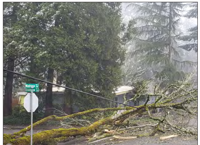
Figure 11. Severe tree damage in mid-Willamette Valley (Wyatt Williams, ODF).
