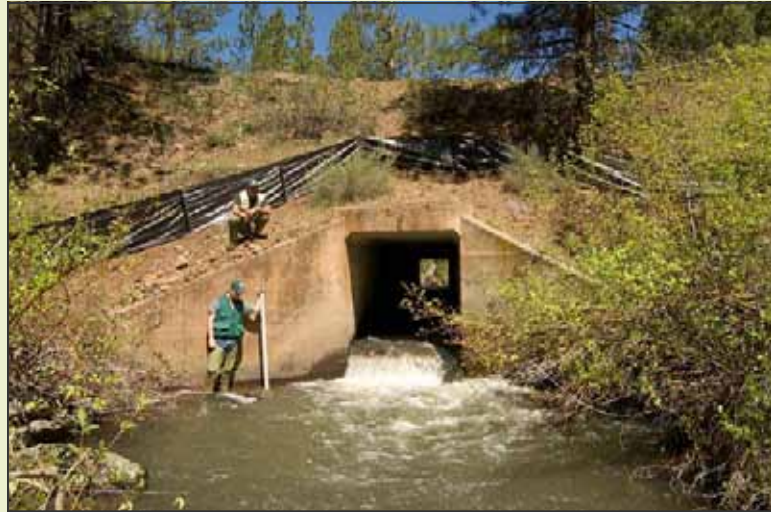
Drews Creek Photo Point #2—Before Restoration This second restoration project on Drews Creek in the Fremont-Winema National Forest shows a culvert that was blocking fish passage underneath the “old” highway before culvert removal.
