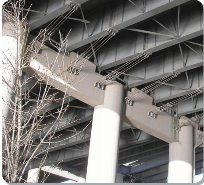
Figure 6.1 : Seismic Retrofit of Marquam Bridge Using Restrain Cables.
