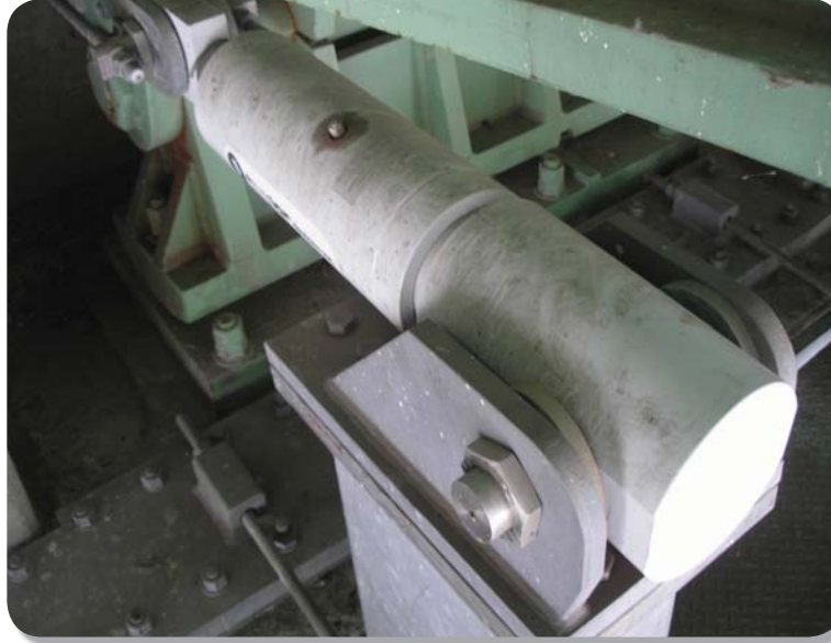
Figure 6.3 : Shock Transmission Units were Installed in Abernathy Bridge as Part of The Seismic Retrofit
