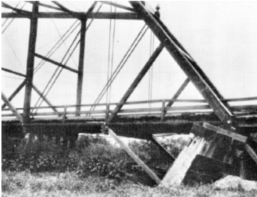
Figure 2.20: South Terminal Pier of Bridge over Salinas River 6.4 km South of Salinas
