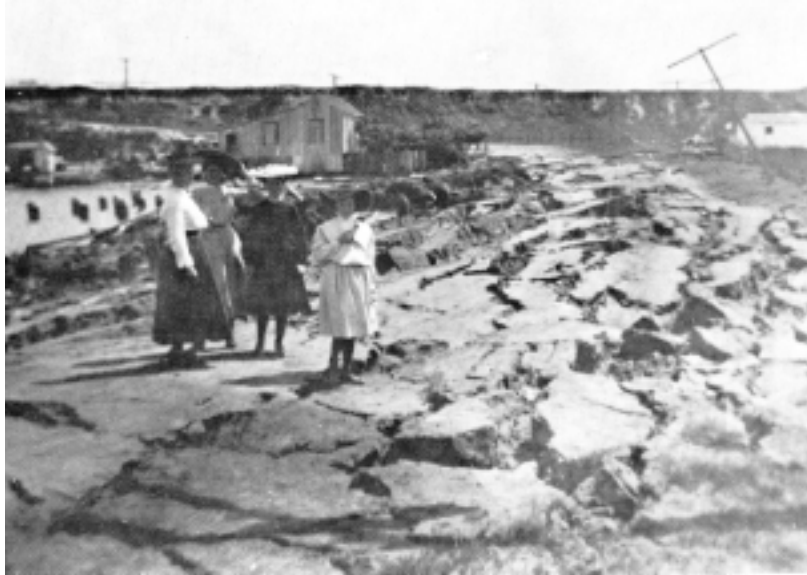
Figure 2.19: Damage from the 1906 San Francisco Earthquake near Monterey Bay
