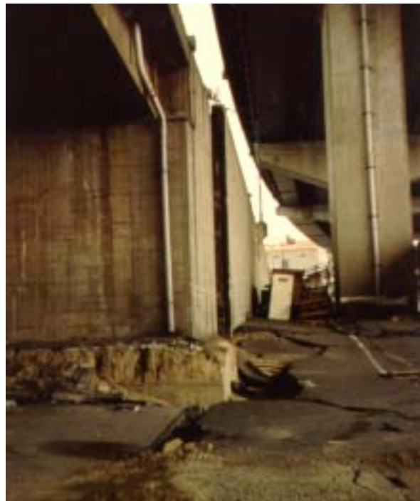
Figure 2.29: Maya Ohashi Bridge
