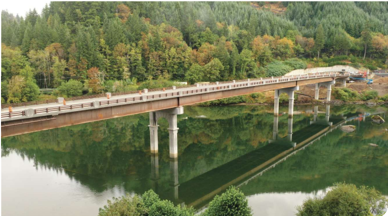
Recently completed Scottsburg Bridge addresses safety concerns. Photo by Bob Grubbs.
