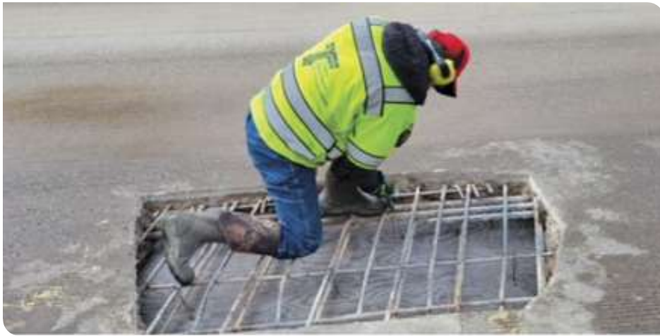
Elk Creek, replacement of damaged deck.
