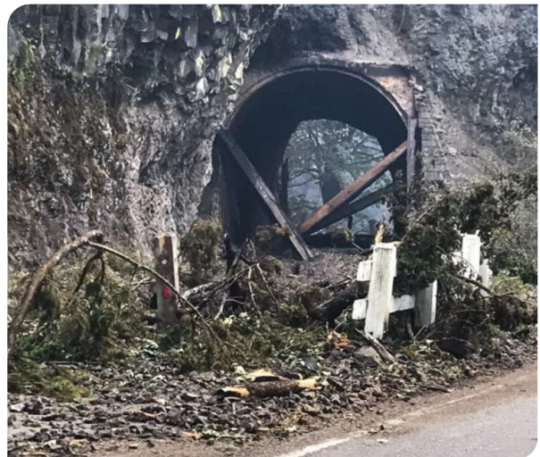
Oneonta Tunnel after 2017 Eagle Creek Fire.
