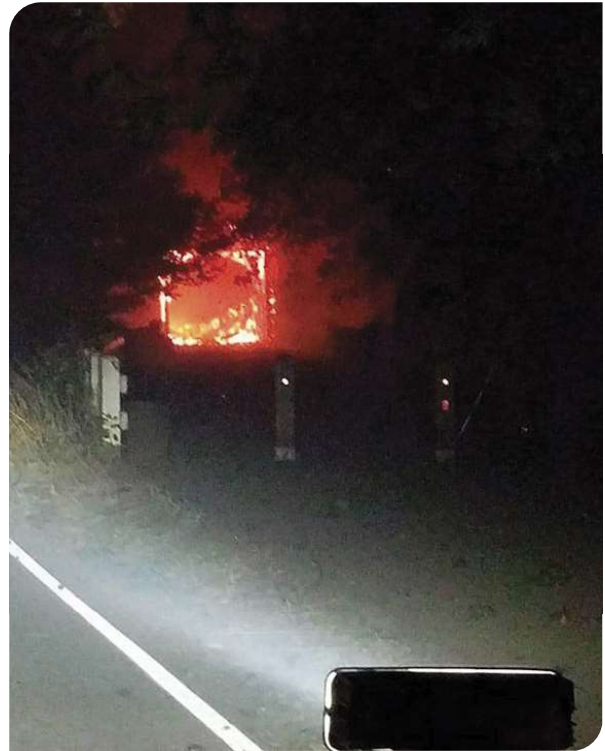
Oneonta Tunnel during the Eagle Creek Fire.
