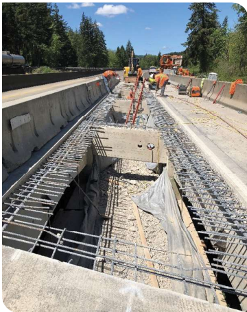
Elk Creek, partial deck replacement work.
