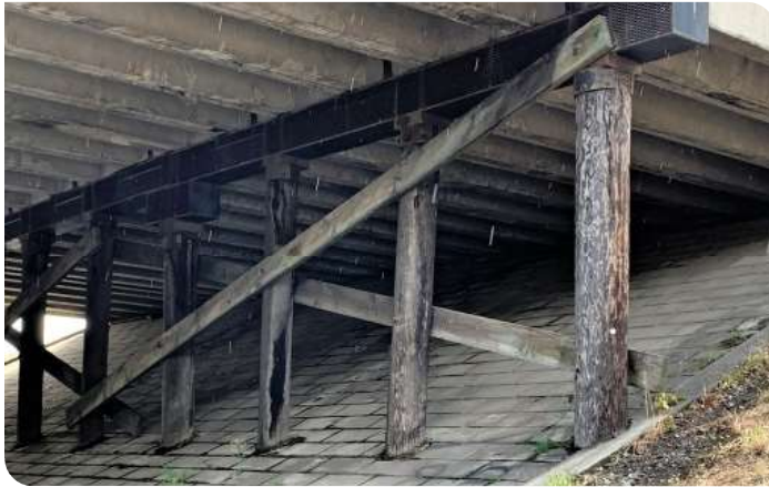
Timber substructure
