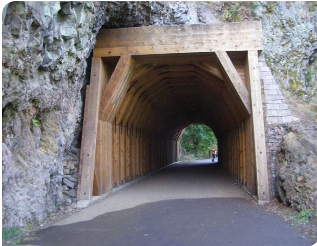
Oneonta Tunnel Prior to Eagle Creek Fire.
