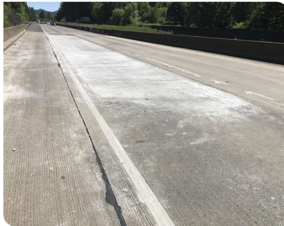
Elk Creek, finished deck repair.
