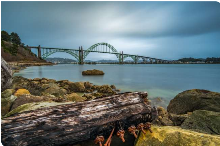
Yaquina Bridge, preservation of steel structure in coastal environment is important to prolong their design life.
