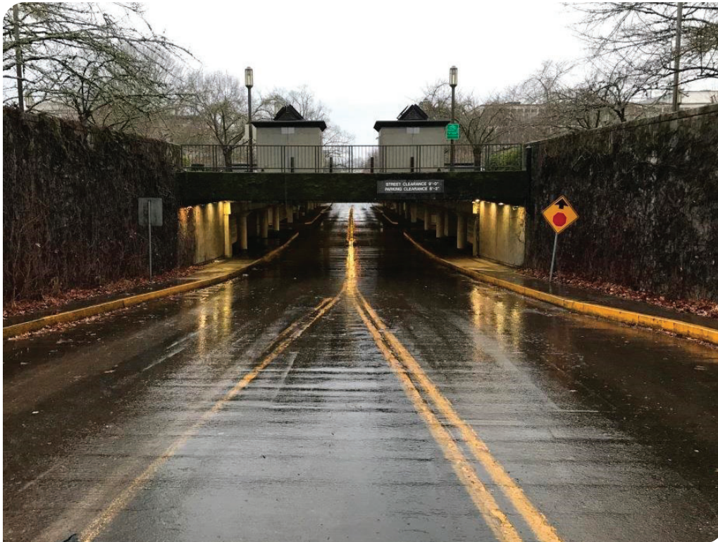
Roadway inside the tunnel accessing the parking area.
