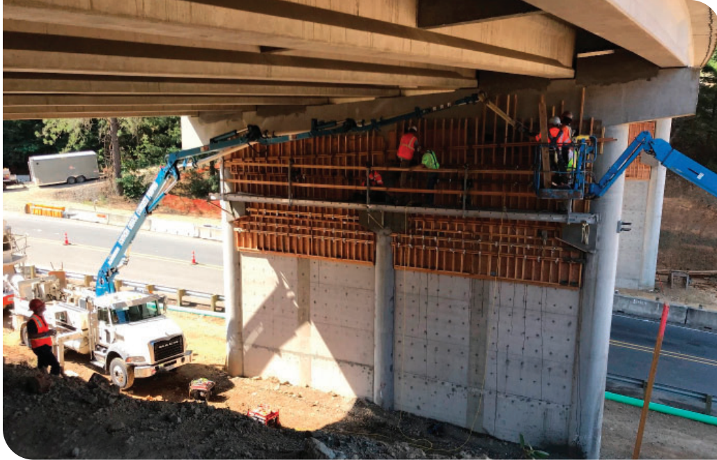
Bent strengthening on Southern Oregon Seismic Bridge Retrofit project.
