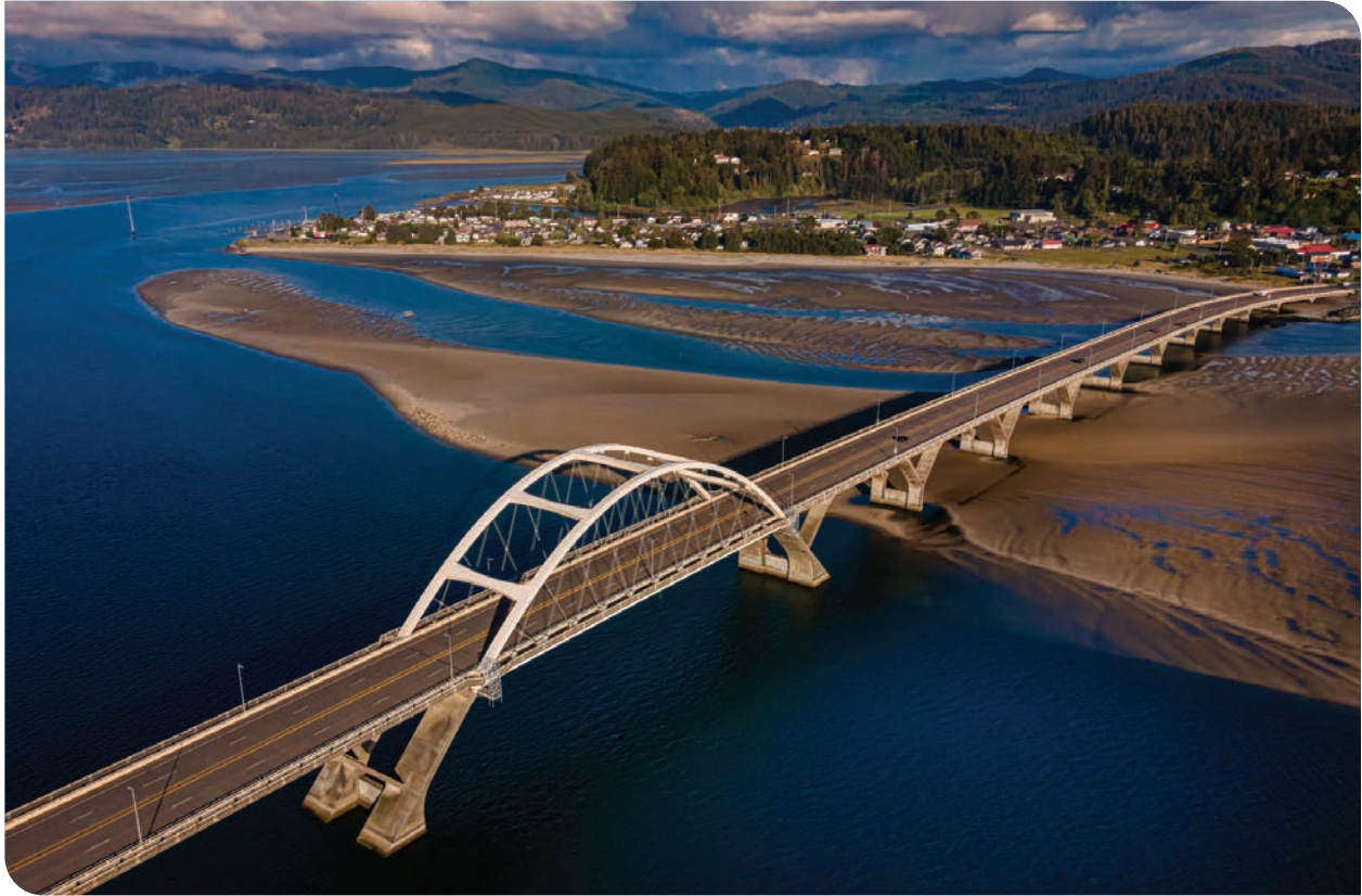
The Alsea Bay Bridge is a major bridge on the Oregon Coast Highway.
