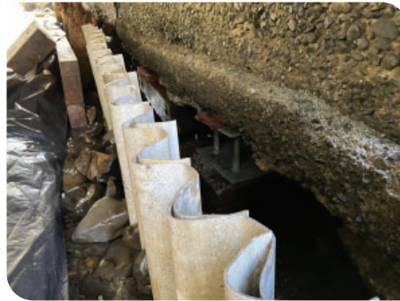
Stay-in place form work placed to protect and support the foundations.
