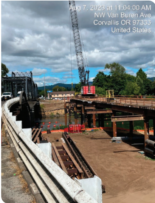
Van Buren Bridge: Temporary structures.
