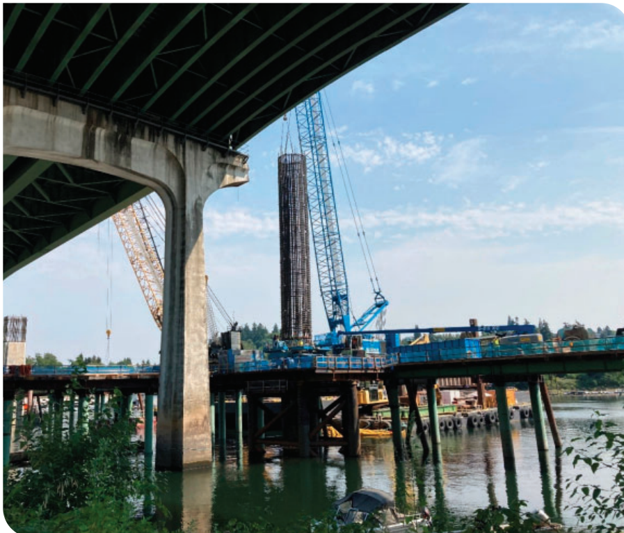
Abernethy Bridge: Construction of new drilled shafts.
