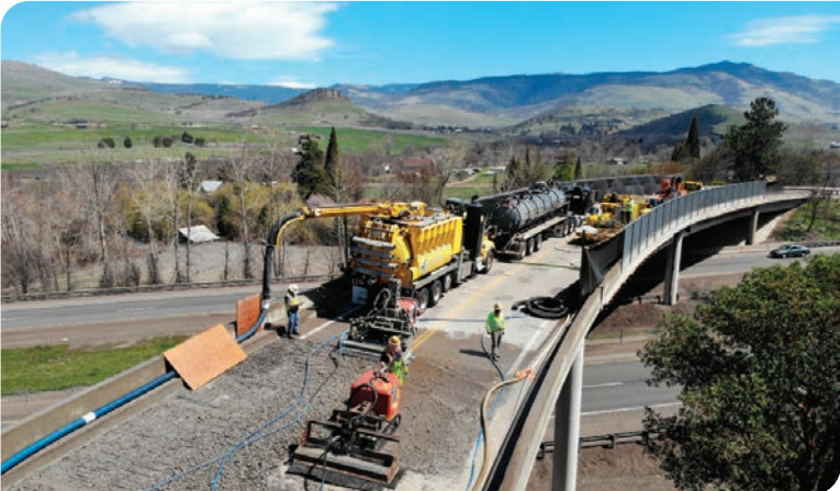
Milling work to remove worn concrete and replace with new surface.
