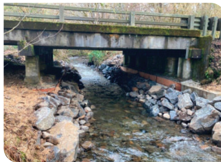
Foundation protected for safe public use.
