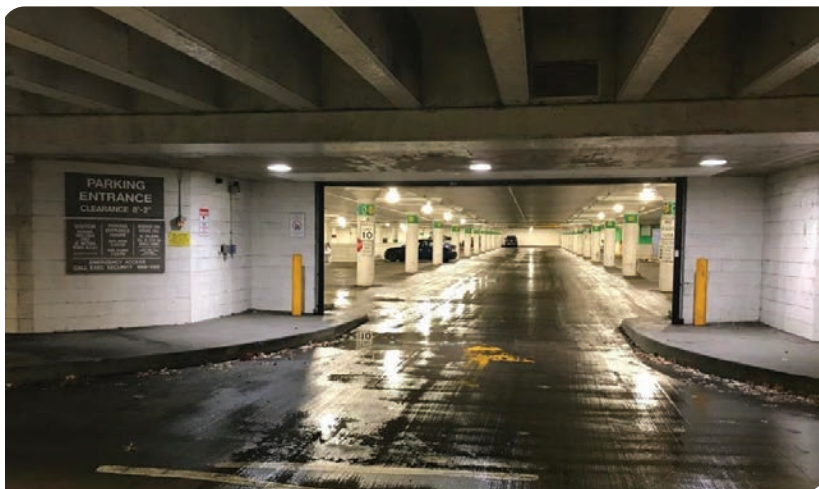
Entrance from tunnel to parking area.
