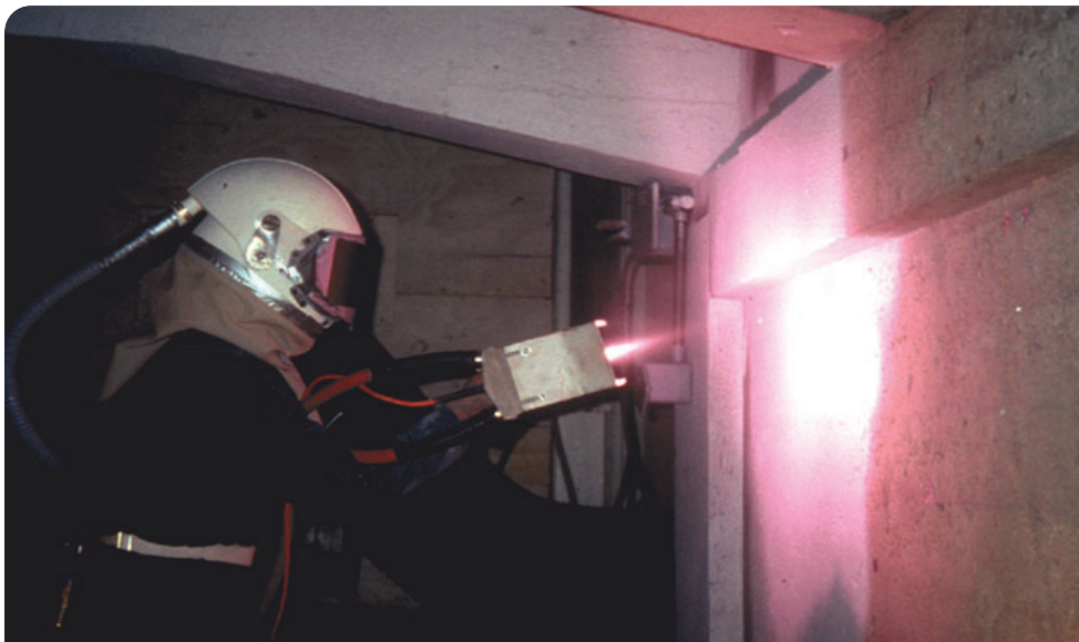
Arc-spraying zinc onto concrete for impressed current cathodic protection system.
