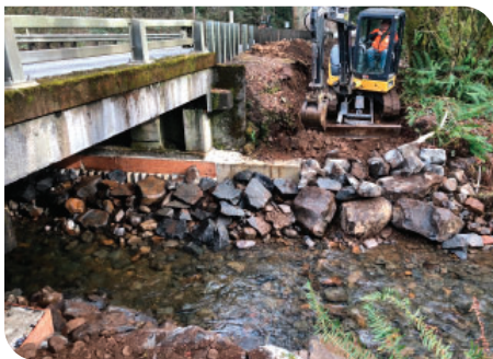
ODOT maintenance crew performing emergency work.
