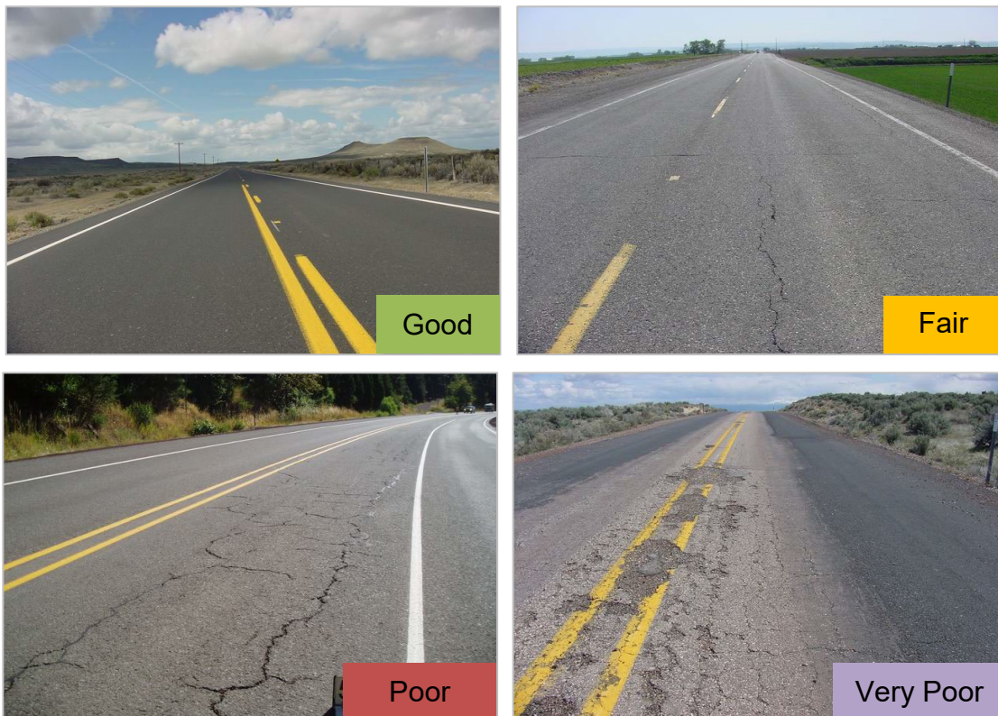
Figure 3 – Example Photos of Pavement – Good through Very Poor
