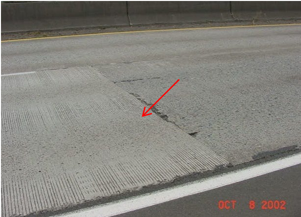
Low – patch is in good condition
