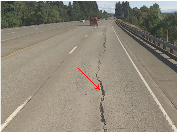
Center – moderate severity (red arrow)
