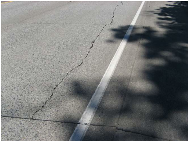
Wheel path – moderate severity
