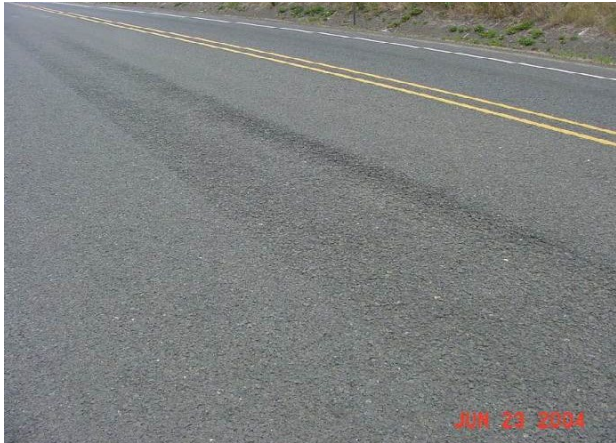
Moderate (both wheel paths, open graded surface)
