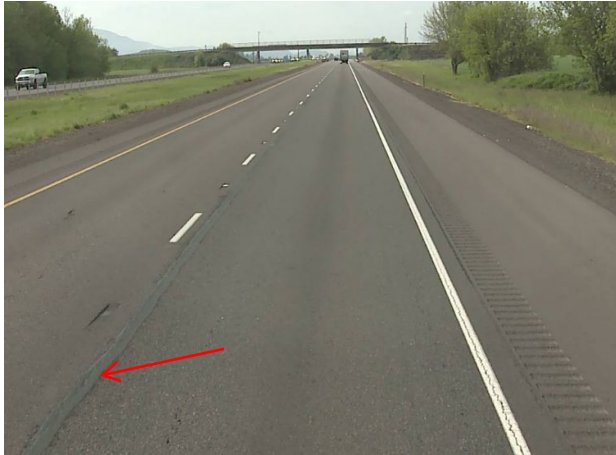
Left edge – sealed severity
