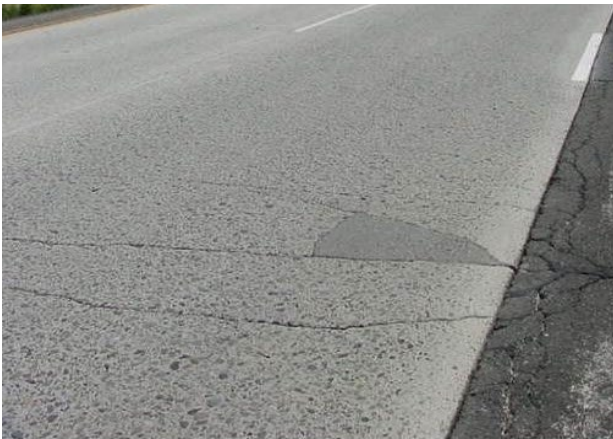
Do not record as a punchout – punchout is completely patched to visible boundaries. Record as patch, not punchout.
