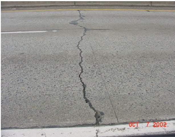
High – transverse crack width is over 1/4"
