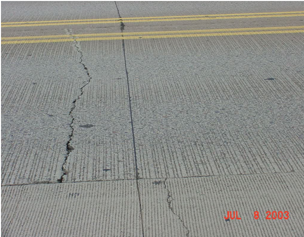
High – transverse crack width is over 1/4"
