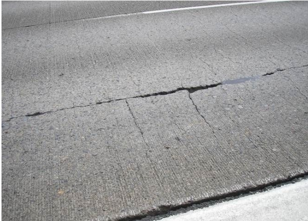
High – right wheel path (based on width)
