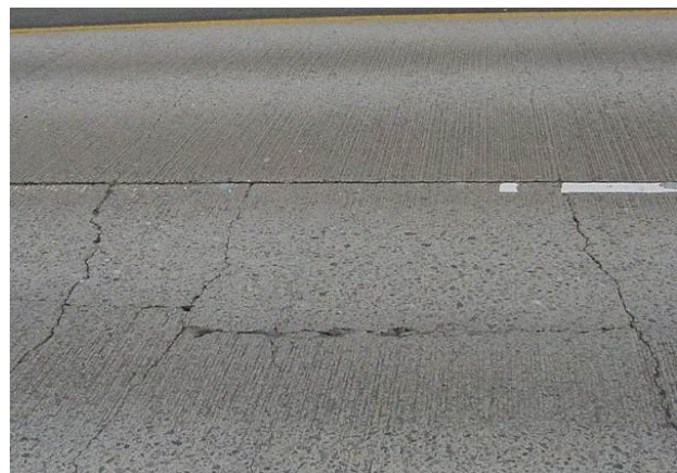
Two low punchouts near centerline
