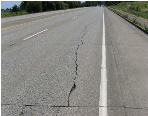
Wheel path – high severity
