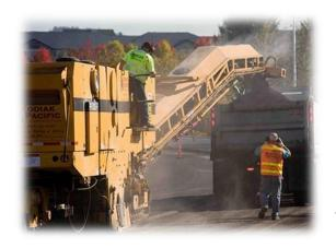
Cold plane pavement removal is used for a variety of treatments including repairing localized failures and removing long segments of highways in preparation for new pavement. Like any construction, a bit of judgment is required to create a good quality milled
