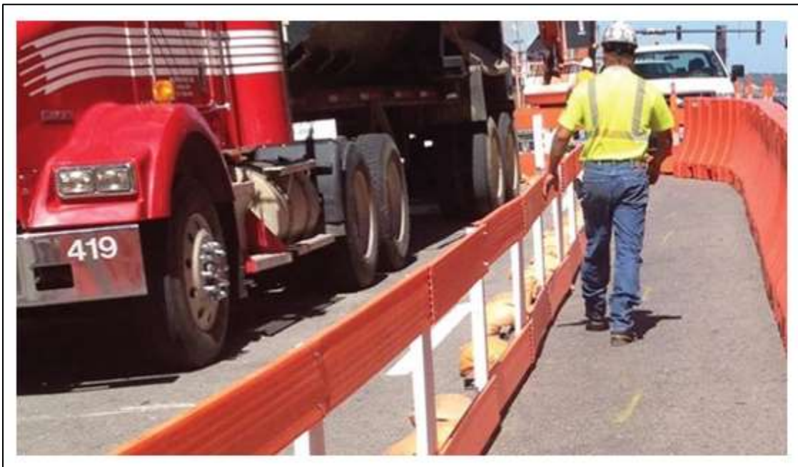
Figure 3-5: PCD between Pedestrians and Work Area
