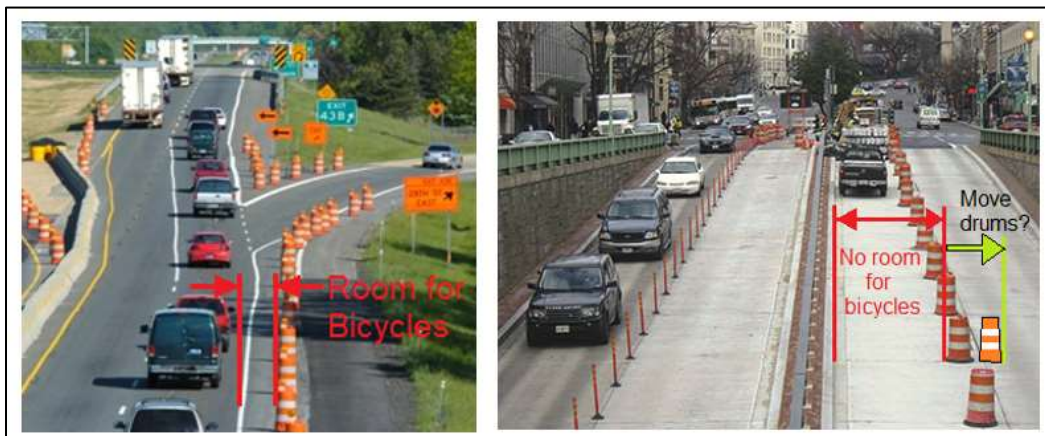
Figure 3-17: Shoulder Width Accommodation for Bicycles
