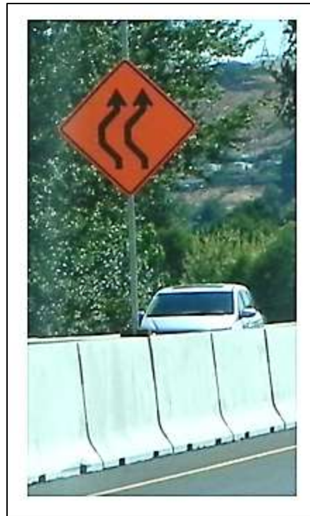
Figure 2-16: Concrete Barrier Sign Support
