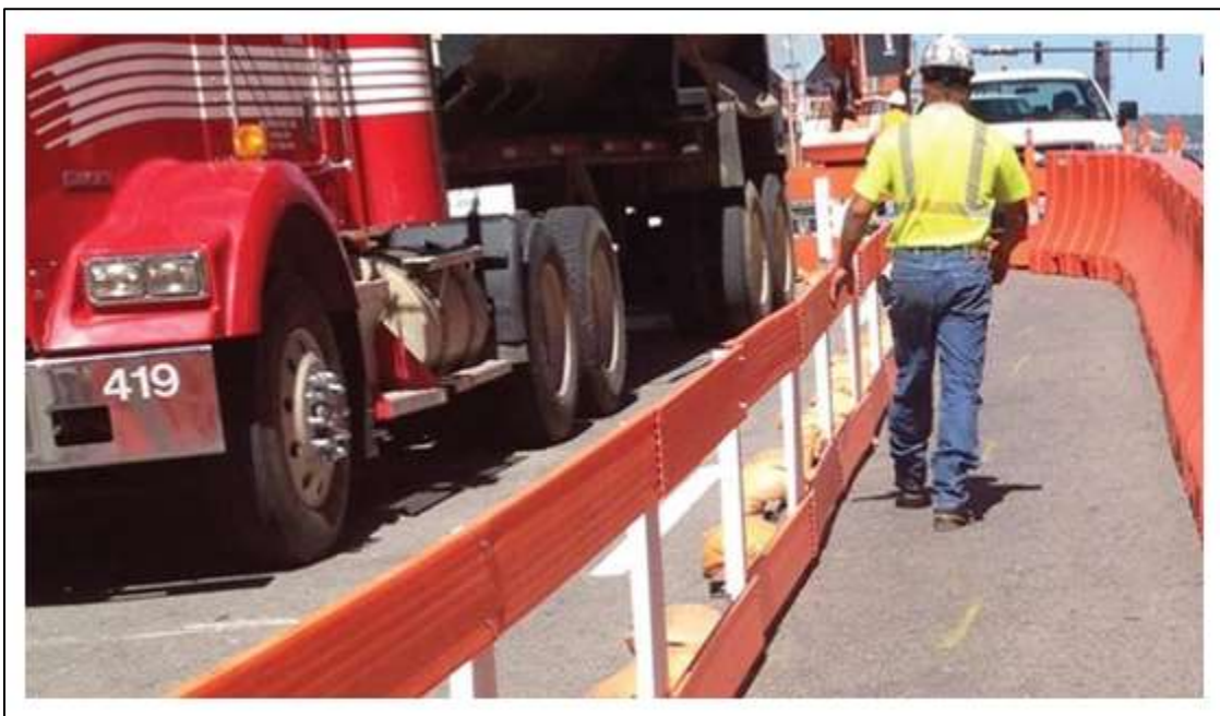
Figure 3-5: PCD between Pedestrians and Work Area
