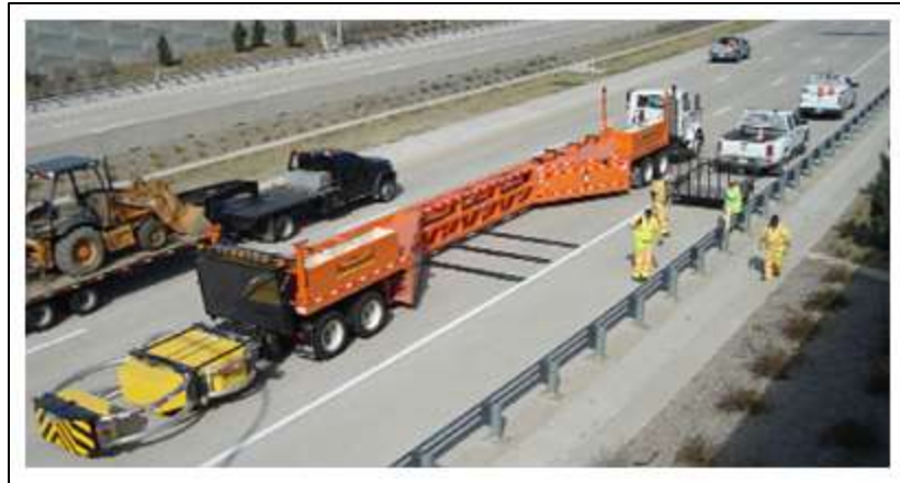
Figure 2-20: Mobile Concrete Barrier
