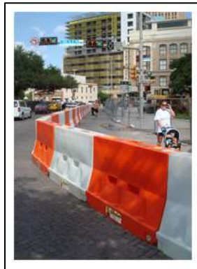
Figure 3-3: PCD between Pedestrians and Vehicles
