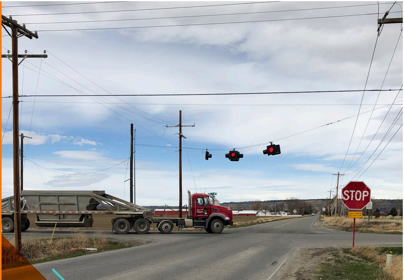
ODOT ARTS Countermeasures I21: Improve Intersection Warning (Larger Signs) and I25: Provide Flashing Beacons at Minor Road Stop Controlled Intersections
