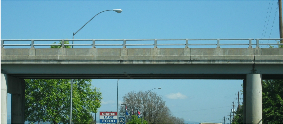
Figure 2.11. “Two Pipe” Variant, Rail Type C/D Medco Lumber Haul Road/Biddle Road Overpass, Jackson County, Oregon Source: Author Photograph, May 2003
