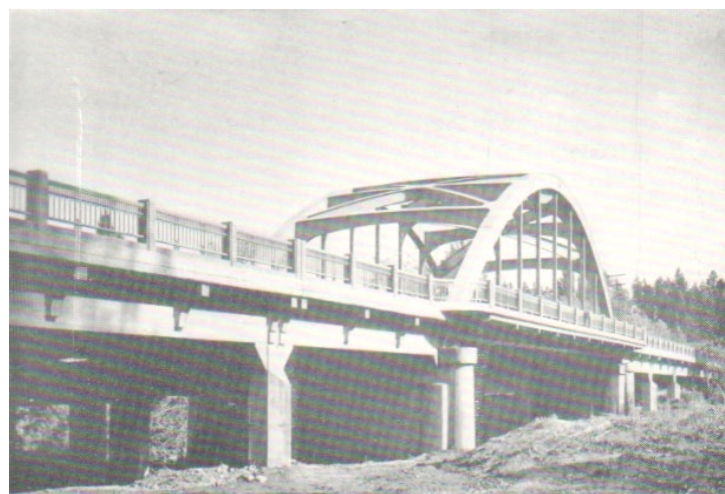
Figure 2.4. Pudding River Bridge, with “Picket Fence” Type Bridge Rail Source: OSHC 18 th Biennial Report (1949:13)
