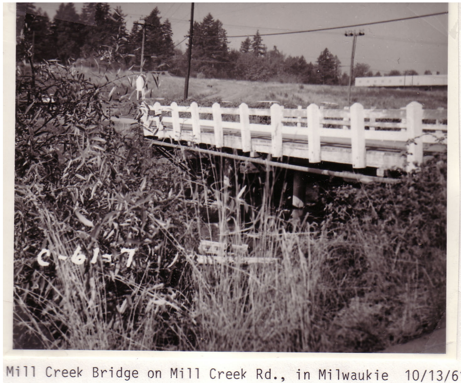
Figure 2.24. Timber Beam Bridge with Typical Wood Bridge Rail Source: ODOT Archive
