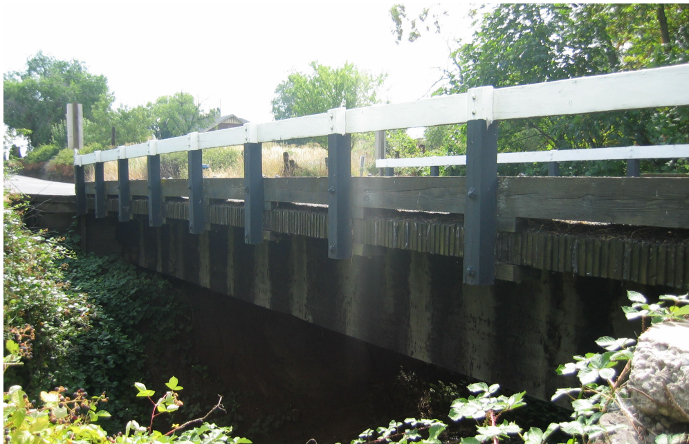
Figure 1.5. Bridge 29C77, Rapp Road at Wagner Creek (Jackson County Bridge No. 57) Timber, Stringer/Multi-Beam Girder (OBI Code #702), 46 feet long, built 1955 Source: Author Photograph, August 2003
