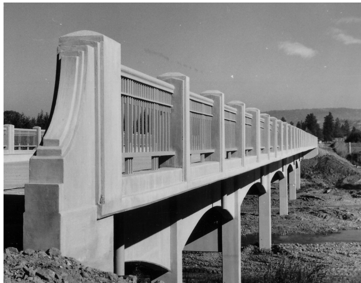
Figure 2.5. Original Picket Fence Bridge Rail and Concrete Transition Detail Isaac Constant Bridge, Central Point, Oregon, 1948 Source: ODOT Archive
