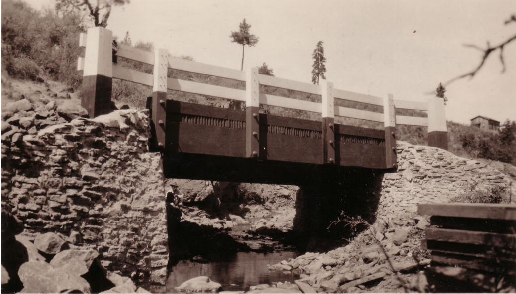
Figure 1.4. Bridge 1084, Timber Stringer Construction (undated), Photo circa 1930 Source: ODOT Archive
