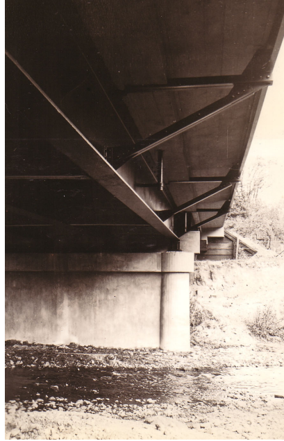
Figure 2.28. “Barbell” Type Piers Supporting a Rolled Steel Beam Bridge with Cantilevered Sidewalks. Benke Bridge, Nehalem Hwy, c1934 Source: ODOT Archive
