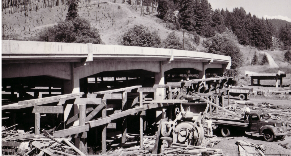
Figure 2.19. Haunched Cast-in-Place Beams, Pacific Highway (I-5) Overpass at Anlauf-Elkhead, Lane County, Bridge #2594, July 1953 Source: ODOT Bridge Files
