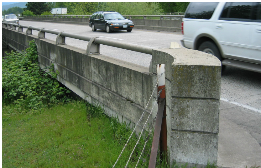
Figure 2.10. One-Pipe Parapet Rail, Bear Creek/I-5 Bridge #8890N, 1962 Source: Author Photograph, May 2003
