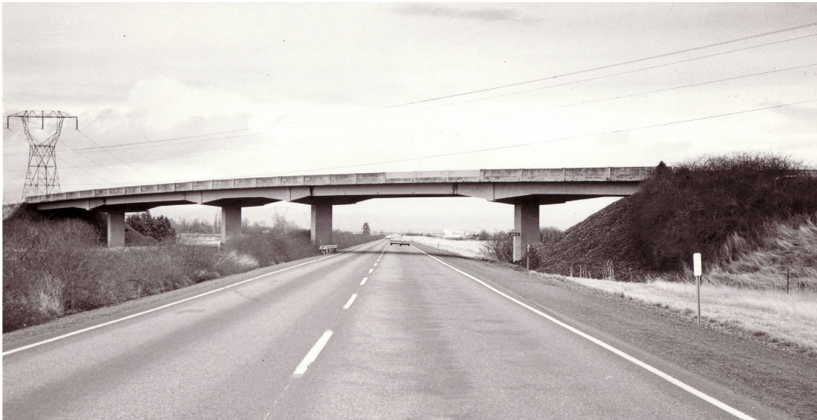
Figure 4.1. Gervais Road Undercrossing, Northbound Interstate 5 Source: ODOT General Files Photo, January 1971
