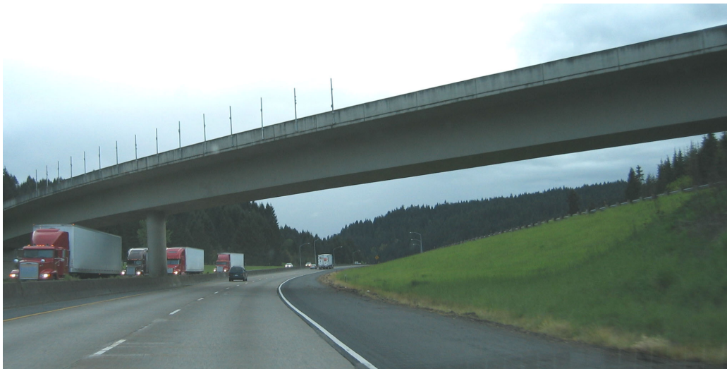
Figure 1.21. Box Girder Overpass on Interstate 5, Douglas County Source: Author Photograph, May 2002
