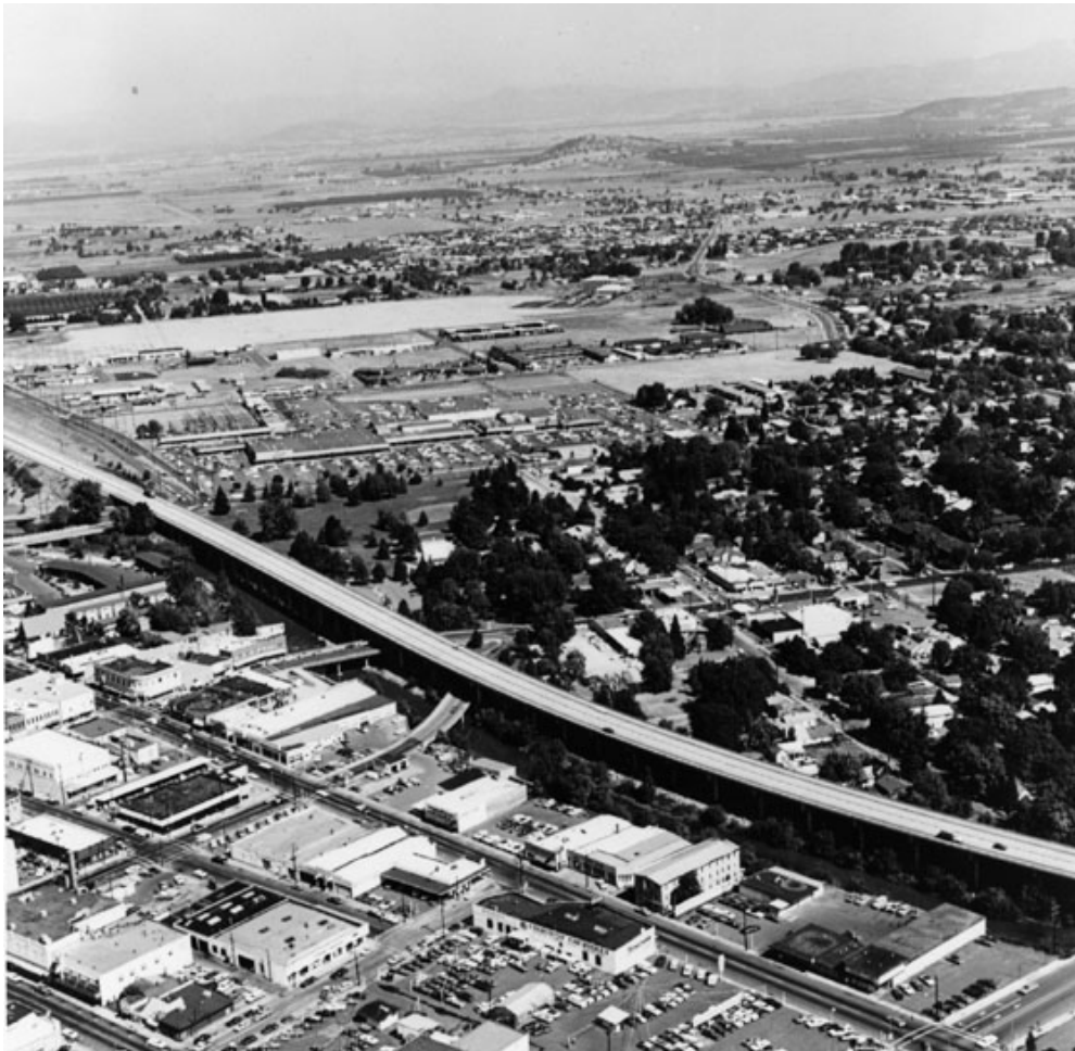
Figure 1.8. The Medford Viaduct, Looking NE over downtown, c. 1963 Source: ODOT Archive
