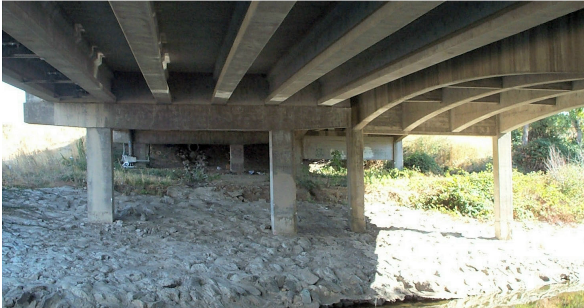
Figure 2.26. Isaac Constant Bridge #697, Central Point, Oregon showing two different variants of square section support piers. (Note pre-stressed I-Beam girders on left, haunched, cast-in-place girders on right.) Source: Author Photograph, November 2002
