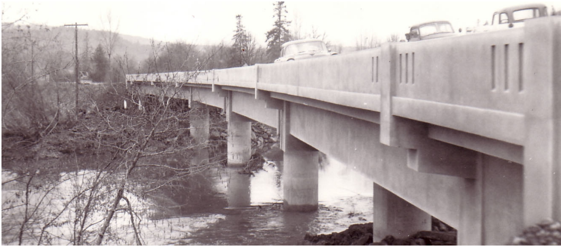
Figure 2.6. “Three Stripe” Bridge Rail, Mohawk Bridge, Lane County, 1958 Source: ODOT Archive
