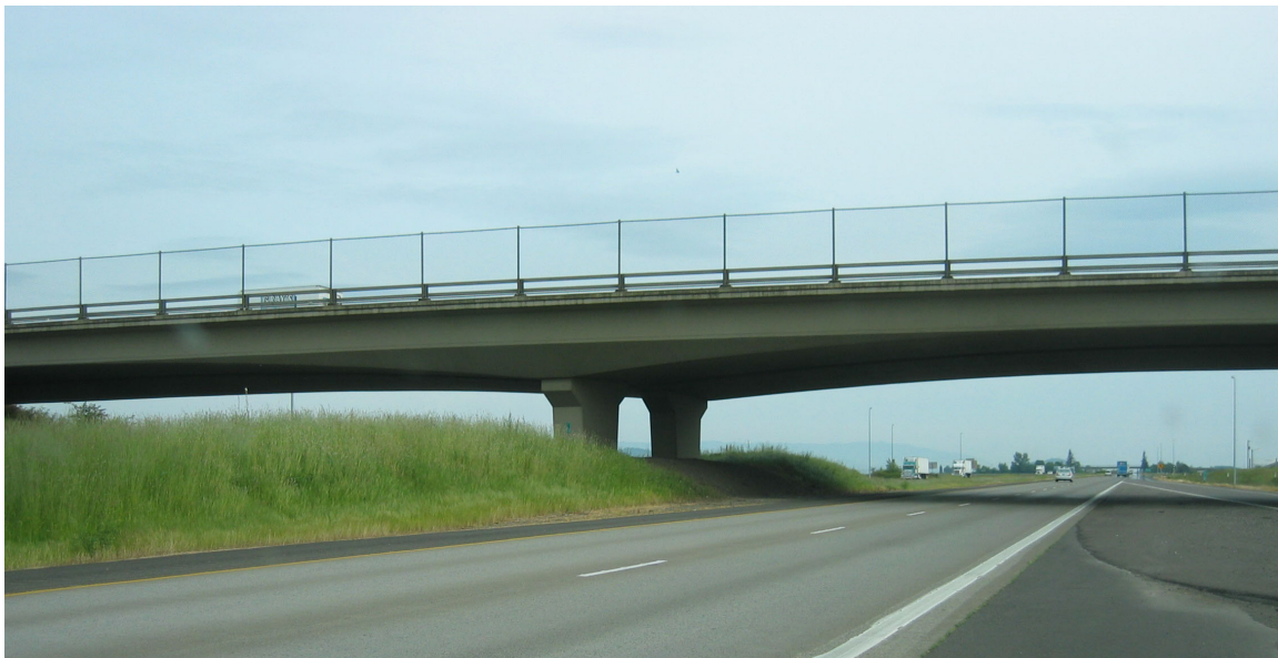
Figure 2.1. Post-1966 Concrete Overpass, Interstate 5, Lane County Source: Author Photograph, May 2003
