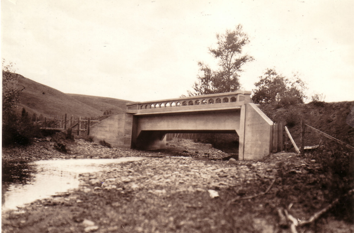
Figure 1.22. Perry Overcrossing, Baker-Unity Highway, Photo Date 1939 Source: ODOT Archive
