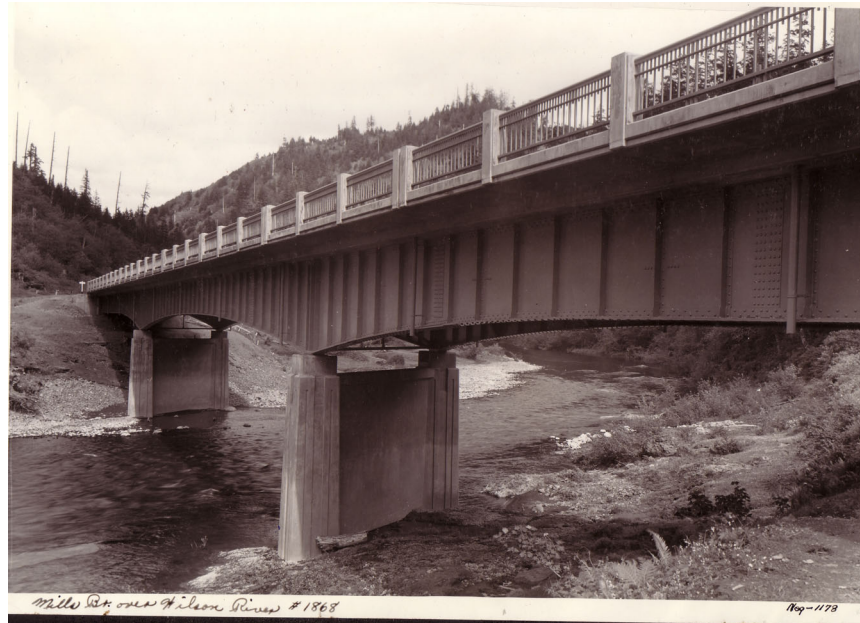
Figure 2.25. Mills Bridge, over Wilson River, (Bridge #1868)
