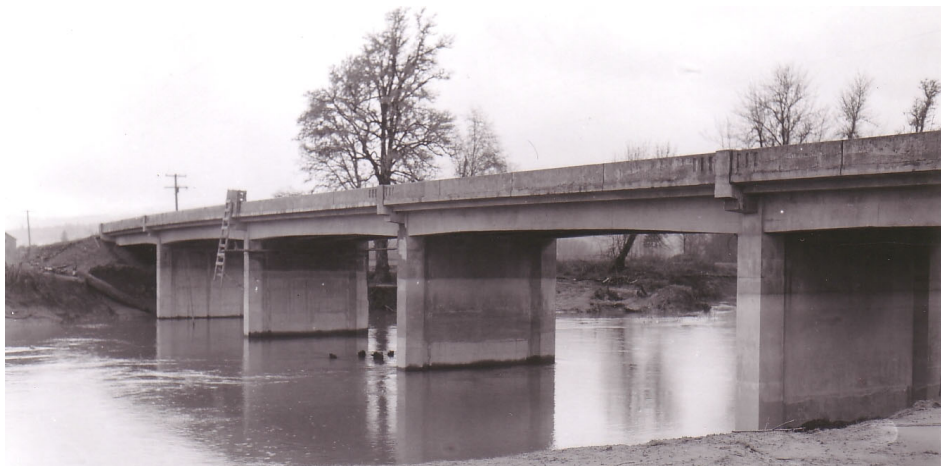
Figure 2.20. Luckimute Bridge from Downstream, February 1956 Source: ODOT Bridge Files
