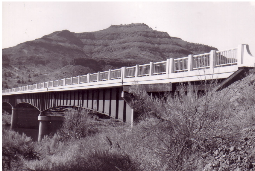
Figure 1.7. Haunched Steel Deck Girder Bridge, John Day Highway, 1955 Source: ODOT Archive
