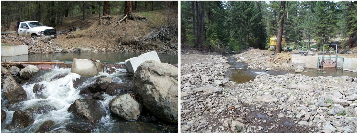
Figure 15: Starveout Diversion Project Before and After
