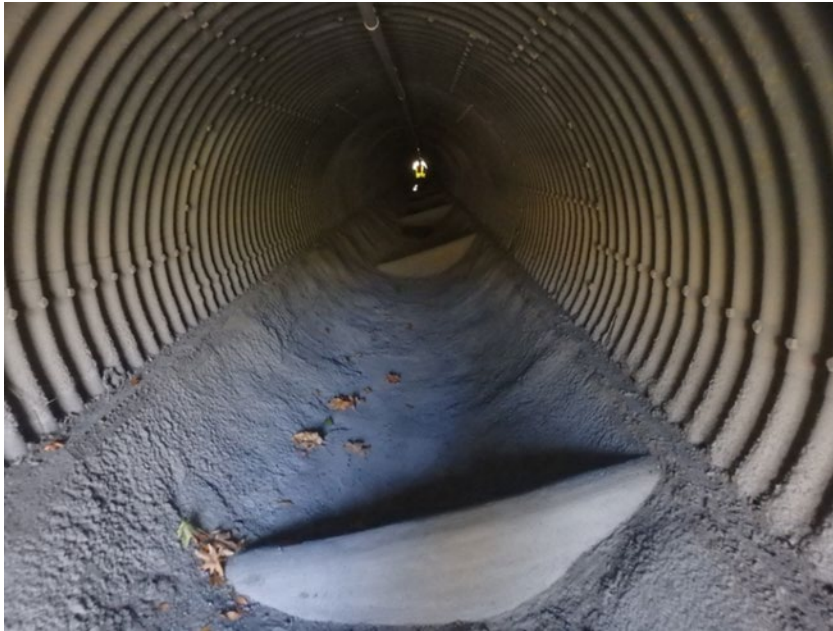
Figure 13: Invert Pave Example
