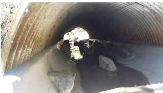
Post-construction - Invert paving and fish rocks installed (9/29/16)
