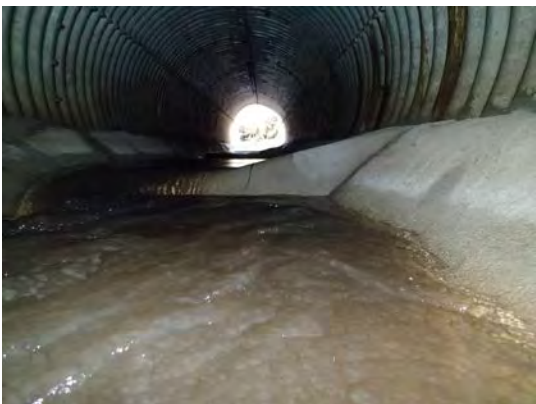
Sloped weir looking upstream toward culvert inlet (10/26/16)
