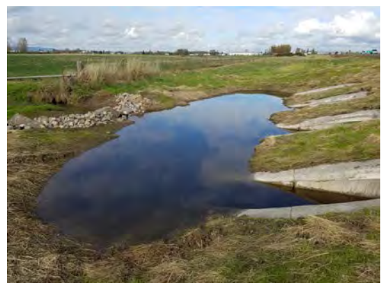
Culvert outlets with weir
