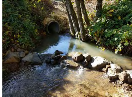
Looking upstream at boulder weir below culvert outlet to back water up into culvert
