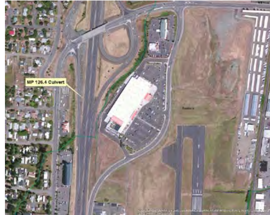
Aerial showing culvert location
