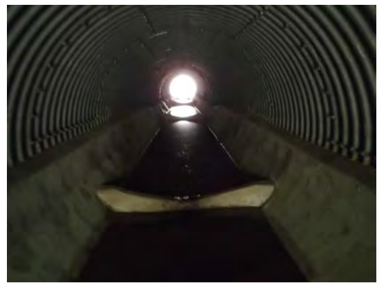
Looking upstream toward inlet
