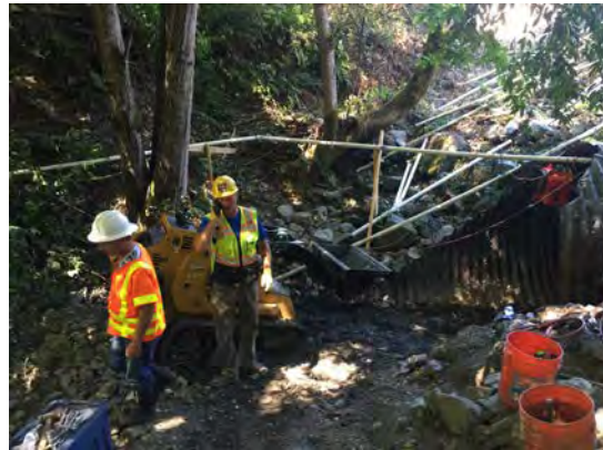
Contractor staging at the inlet of culvert (8/5/16)
