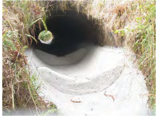
Culvert outlet showing invert paving and weirs
