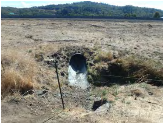
Inlet of culvert upstream of I-5 (9/20/16)
