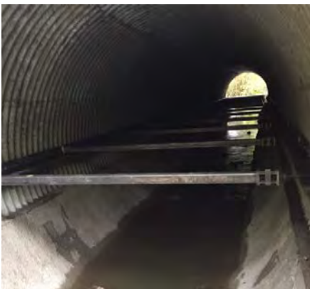
Post-construction bracing and invert paving (10/20/16)
