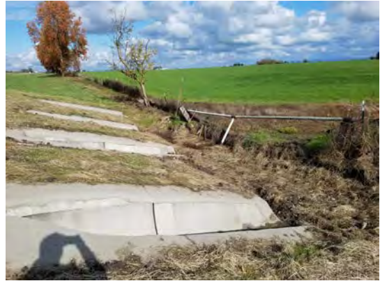
New culvert inlets
