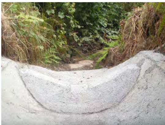
Culvert outlet looking downstream showing weir
