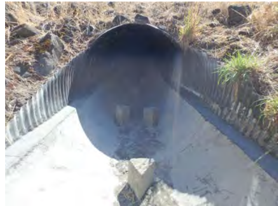
Close-up of inlet of culvert upstream of I-5 (9/20/16)
