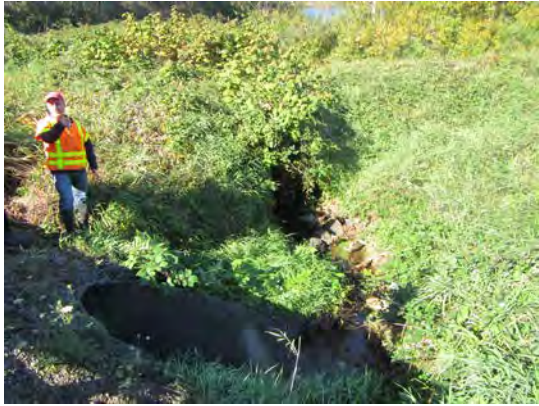
Culvert outlet looking downstream toward boulder weir
