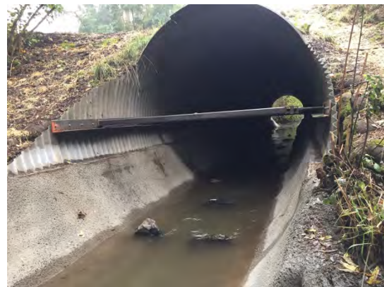
Post construction fish rocks (10/20/16)
