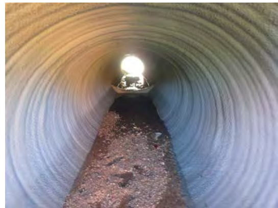
Inside of culvert showing centrifugally cast concrete liner
