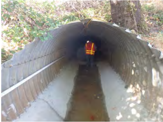
Walking into culvert inlet right post-construction (9/20/16)
