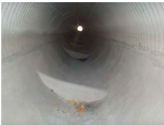
Invert paving with sloped weirs prior to the return of flow (9/20/16)
