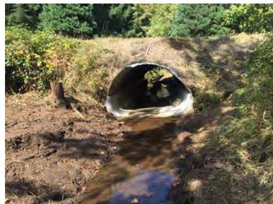
Post-construction looking upstream at the outlet (9/29/16)
