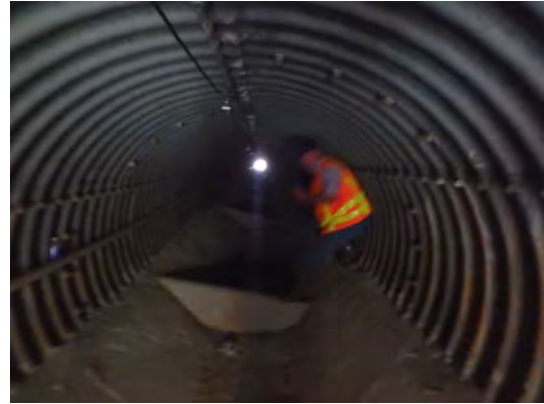
Sloped weirs prior to re-watering of culvert (9/20/16)
