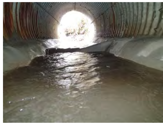
Sloped weir looking upstream toward culvert inlet (10/26/16)
