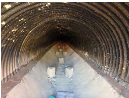
Inside culvert showing invert paving and roughness features (9/20/16)
