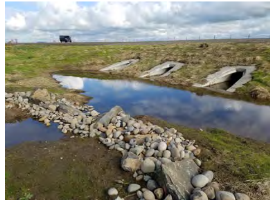
New downstream weir to back water into culverts
