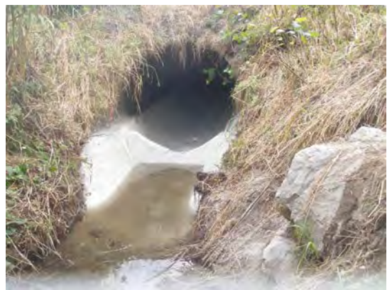
Inlet of culvert flow returning to creek
