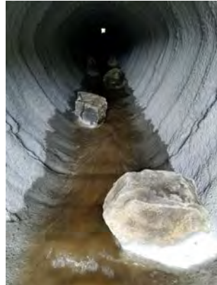
Inside culvert showing fish rocks and centrifugally cast concrete
