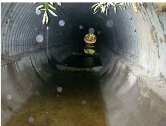
From outlet looking upstream toward inlet
