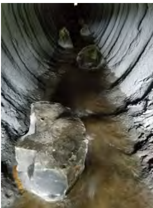
Fish rocks inside culvert
