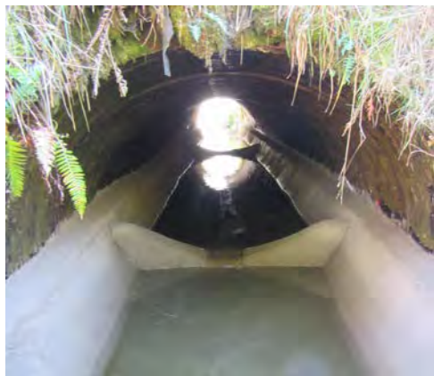
Inside Culvert showing flow returning to creek
