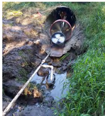
Outlet of culvert during construction showing work area isolation
