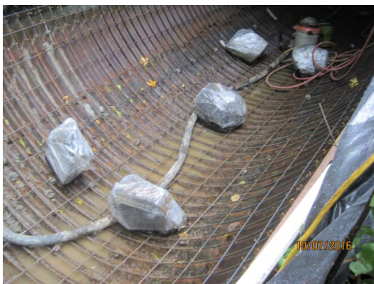
Rebar cage and fish rocks in place prior to invert paving (10/7/16)
