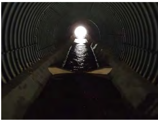
Looking downstream toward outlet
