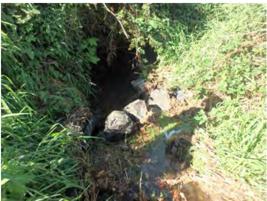
Downstream rock weir to back water up to culvert outlet
