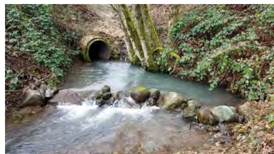
Downstream weir at winter base flow – February 2018
