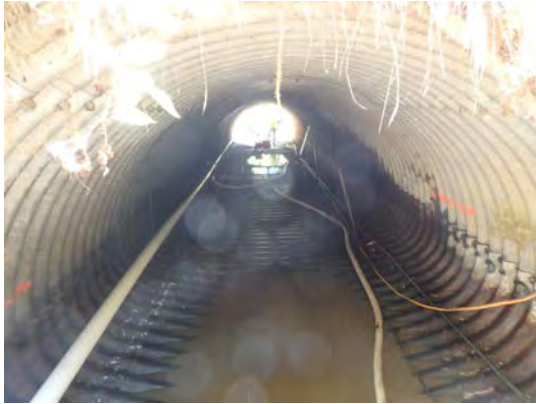
During construction dewatering and cleaning out the culvert (9/20/16)
