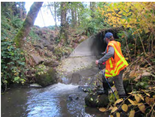
Looking upstream at culvert outlet - fall 2017
