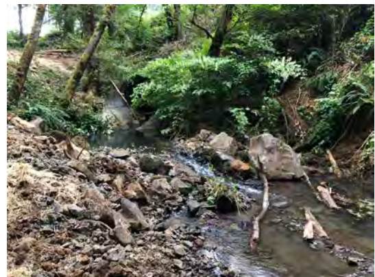
New downstream weir to back water up into culvert. Installed summer 2018
