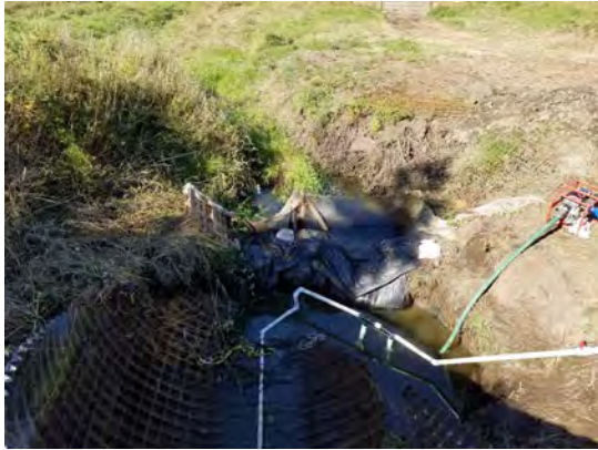
In-water work area isolation at culvert inlet - 2017
