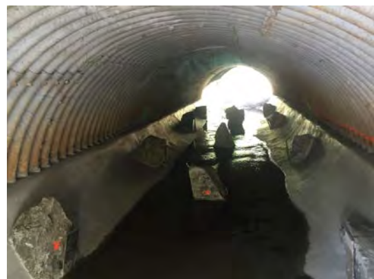
Post-construction - Invert paving and fish rocks installed (9/29/16)
