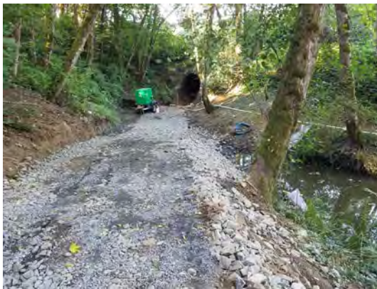
Looking toward culvert outlet and access road - 2017.
