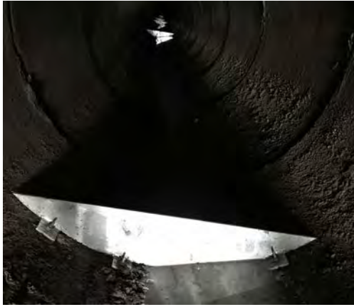
Internal culvert baffles
