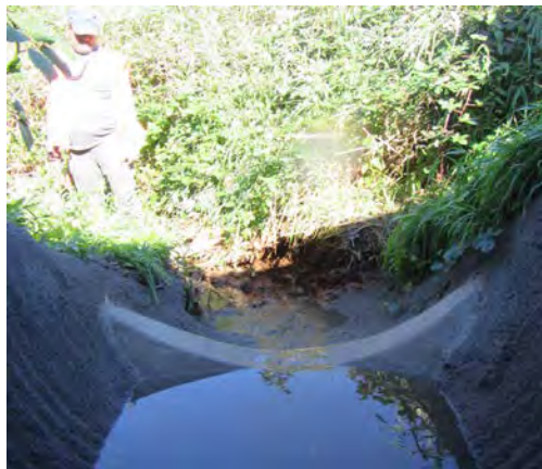
Looking downstream at outlet of culvert
