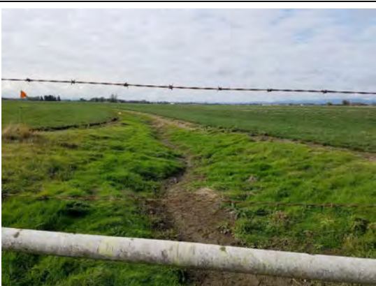
Looking upstream at inlet side of culvert
