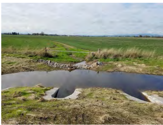
Looking downstream from outlets
