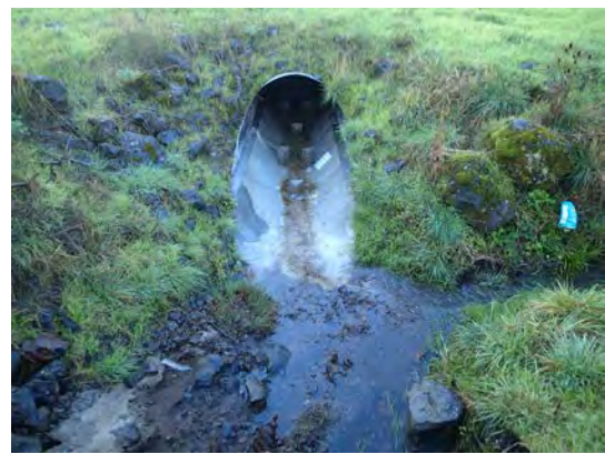
Inlet of culvert with flow (10/26/16)
