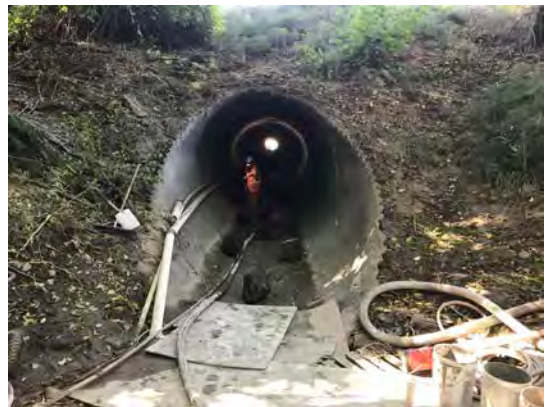
2018 construction - placing fish rocks
