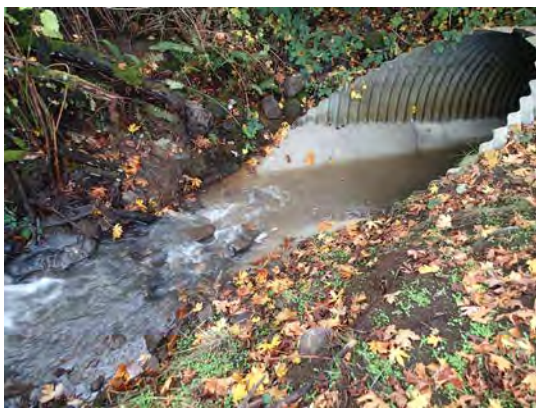
Culvert inlet post-construction (10/26/16)
