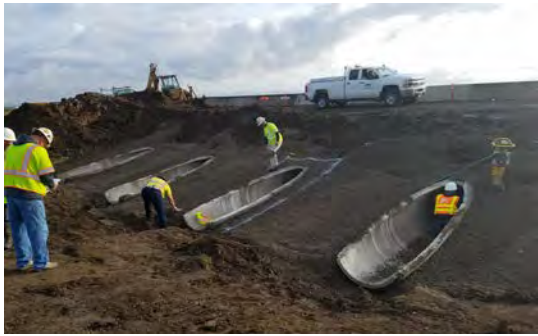
New culvert outlets in construction
