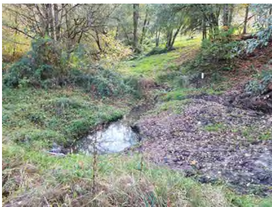
Looking downstream at outlet of culvert
