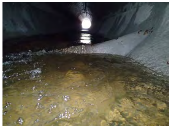
Typical sloped weir configuration with low flow (10/26/16)
