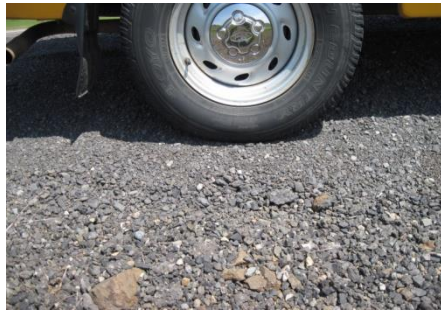
Compacted Grindings on Road Shoulder
