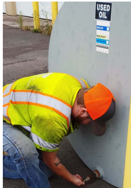
Check the inspection port to determine if liquids are present between the double-walls of the tank.
