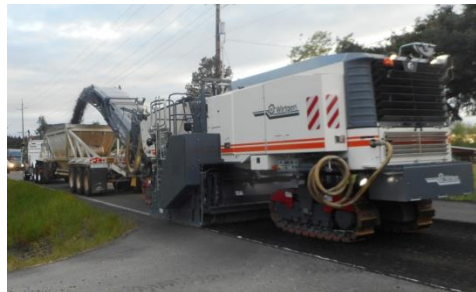
Asphalt Grinding Equipment
