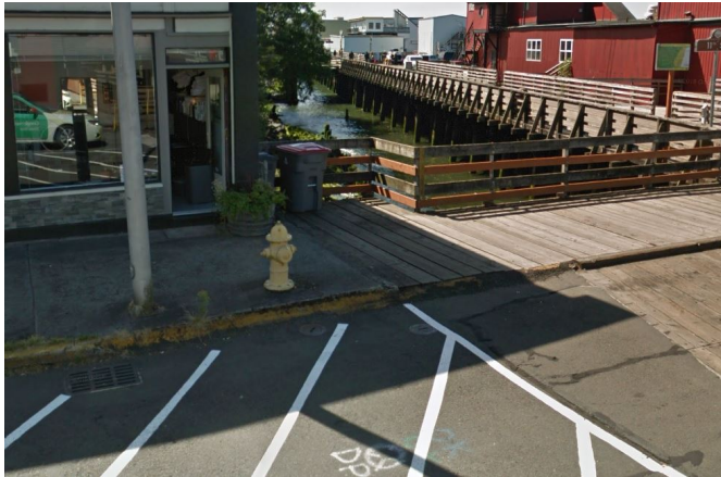
Figure 18: Wood Sidewalk = OTHER.
