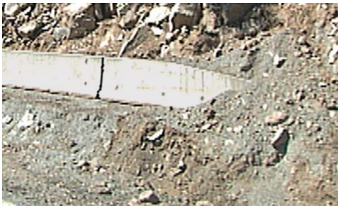
Figure 8: Buried in Back Slope (BIBS) - End is buried into the slope of the land (i.e., side of hill).
