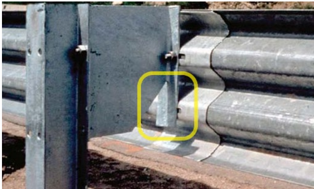
Figure 66: MOD THRIE (Modified Thrie) - Characterized by the notch in the block-out.
