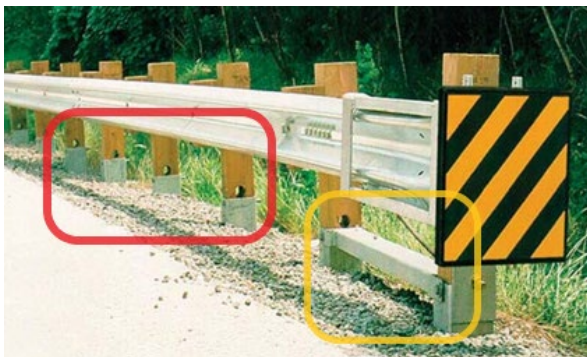
Figure 14: ET 2000 - Has a flat end that is perpendicular to the road. All posts are drilled to breakaway; and there is a ground strut. ET 2000 has a square end.
