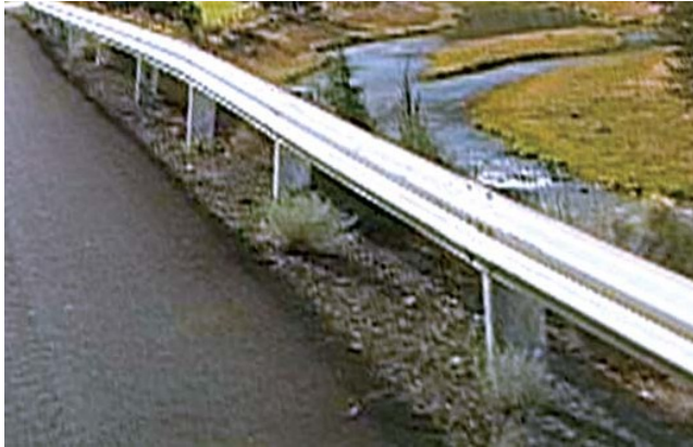
Figure 65: FLYING W - Characterized by a “wing” on each side of the guardrail; hence the name.
