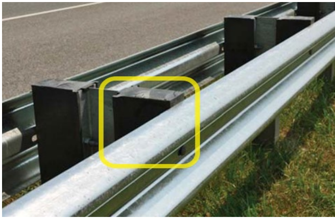
Figure 81: Steel Posts with Plastic block-outs (black polycarbonate).
