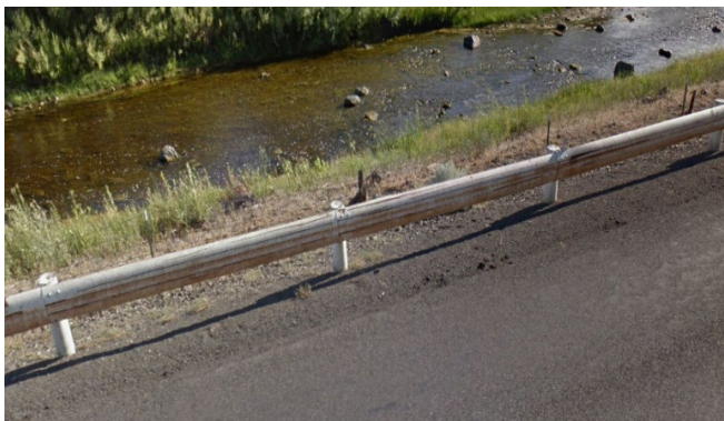
Figure 67: HALF MOON - The rail is shaped like a half-circle. It does not have the typical ridges other guardrails do.
