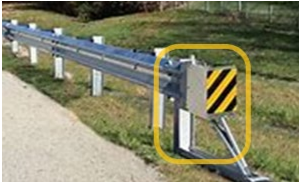
Figure 5: Image of terminal
