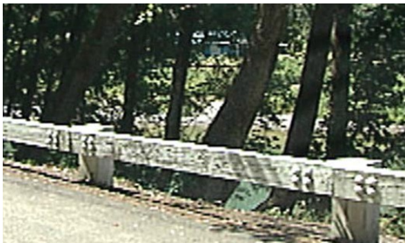
Figure 69: SBT (Steel Backed Timber) - Rectangular prism shaped timber with steel backing.
