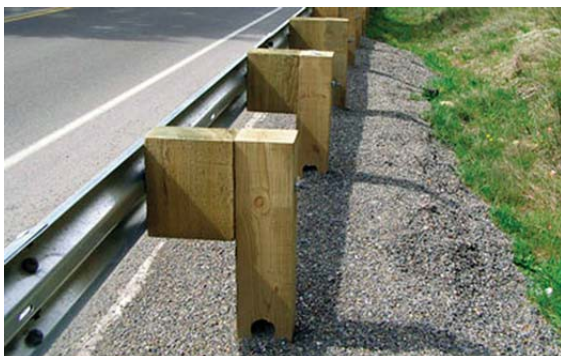
Figure 80: Wood Posts with wood block-outs.
