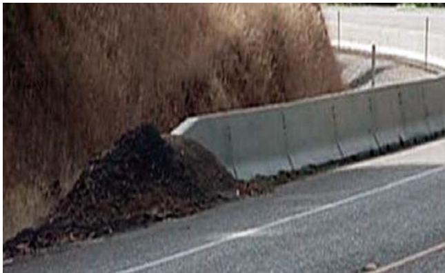
Figure 7: Mound - End is buried in a man-made mound of earth.
