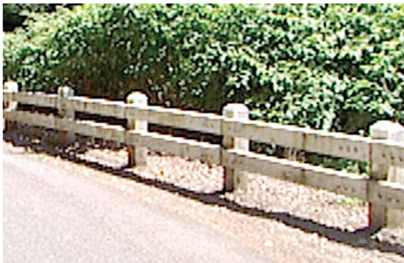
Figure 70: TWO RAIL SBT (Two Rail Steel Backed Timber) - Two wooden rails painted white with steel backing.
