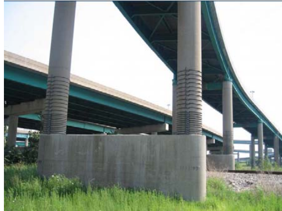
Figure 5.10: External prestressing steel retrofitting of columns in Illinois
