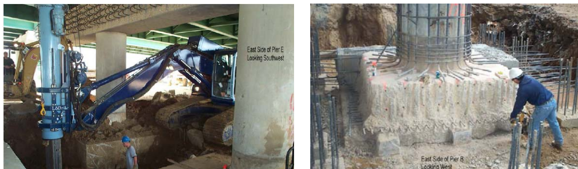
Figure 5.6: Footing overlay on Hernando-Desoto Bridge (photo: R.A. Imbsen)
