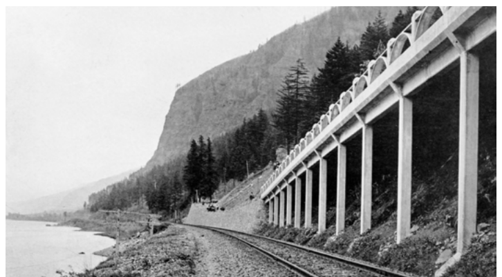
Historical image of the west viaduct next to rail line. Photo courtesy of the David Sell Collection
