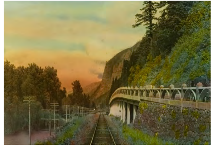
Historical image of the west viaduct next to rail line. Photo courtesy of the David Sell Collection
