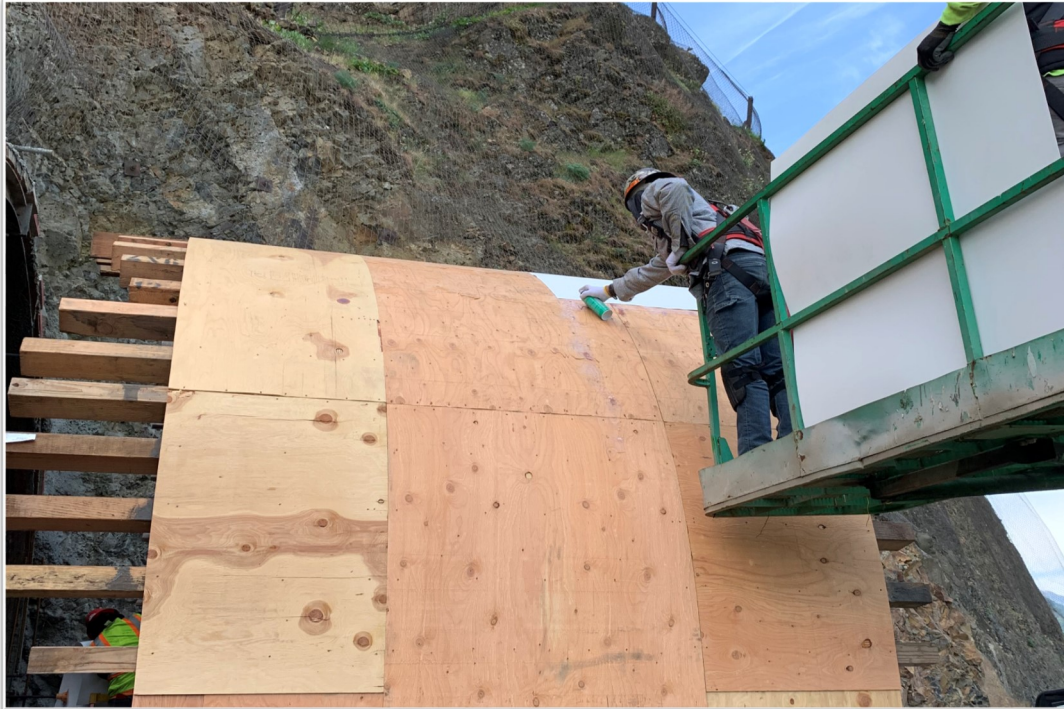
West Portal Concrete Structure Support Assembling
