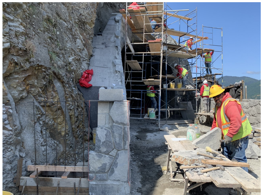
Stone Masonry on Façade at East Portal of Tunnel
