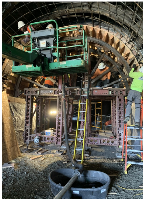
Concrete Pouring at West Portal Arch
