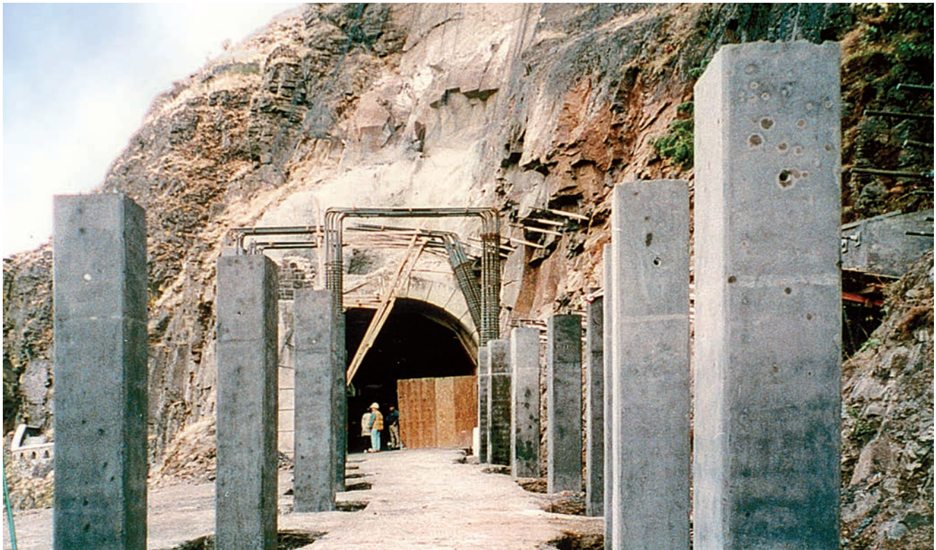
Figure 110—Rockfall Catchment Structure During Construction
