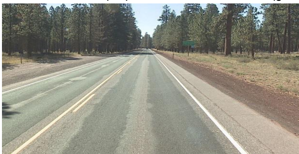
State – Rut Patches (fair) National – No rut or crack (good)
