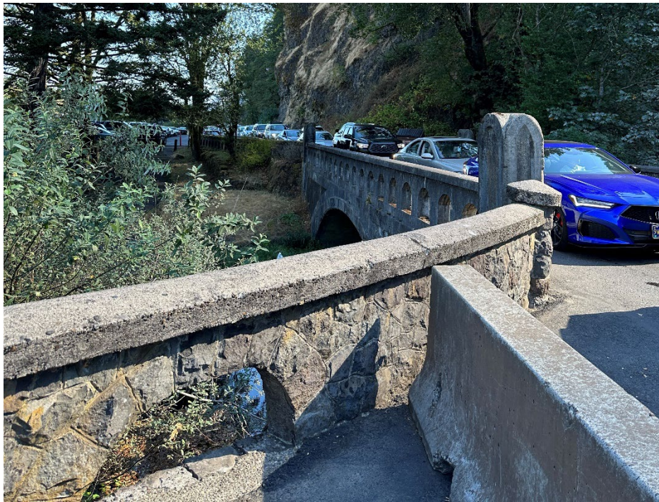
Figure 6-1. Vehicle Queue and Congestion on the Historic Highway at Multnomah Falls Monday, September 26, 2022.
