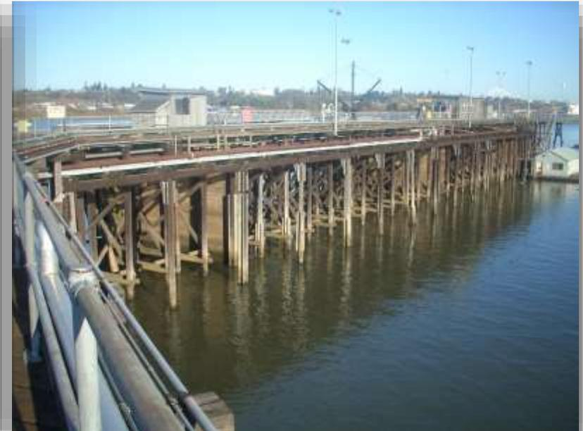
Marine docks receiving fuel will be damaged with moderate earthquake
